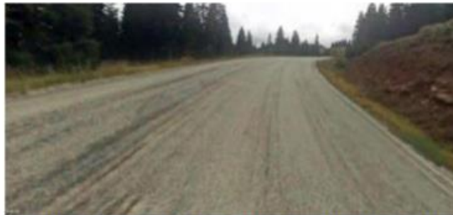
Figure 1: A curve on this segment of the Ogden River Scenic Byway (SR 39) without delineation or barriers (Google).
