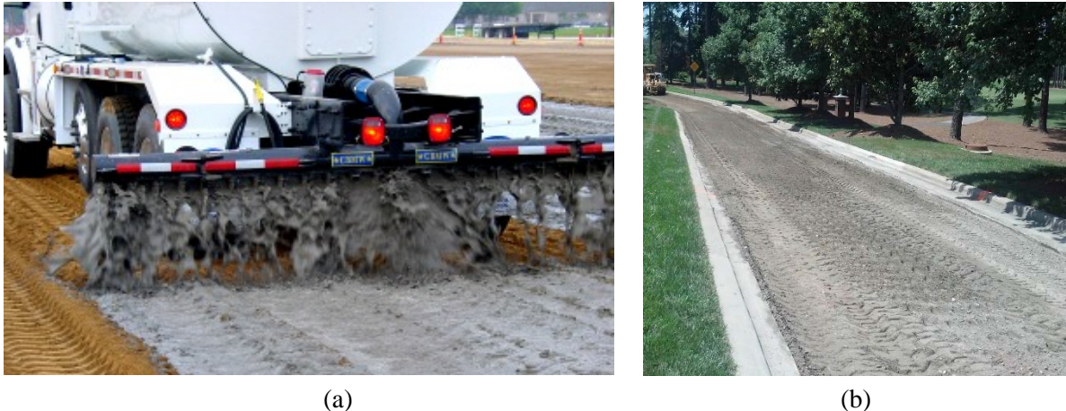
Figure 5-22: (a) Slurry Mixing and (b) Dry Powder Mixing in the Field.
