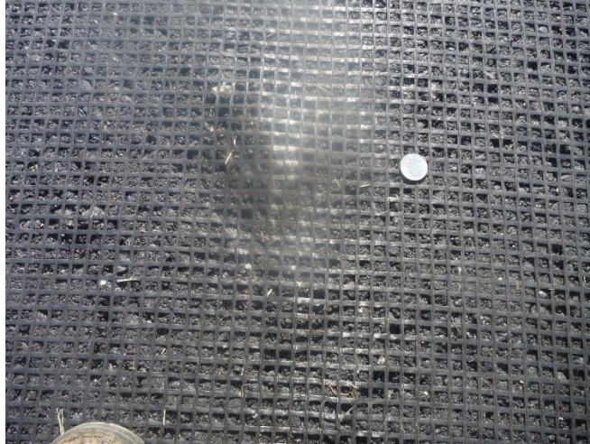
Figure 8. Interlayer Used on US 460
