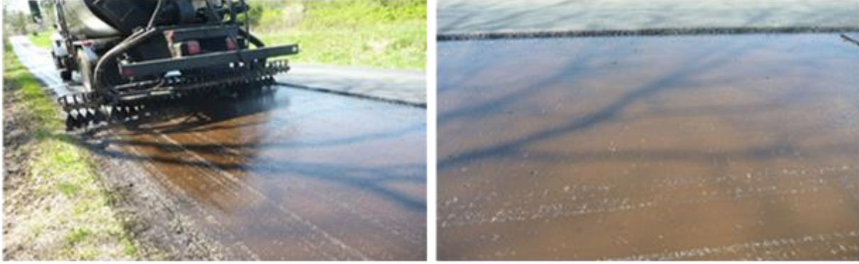
Figure 5. Tack Application at the Control Section
