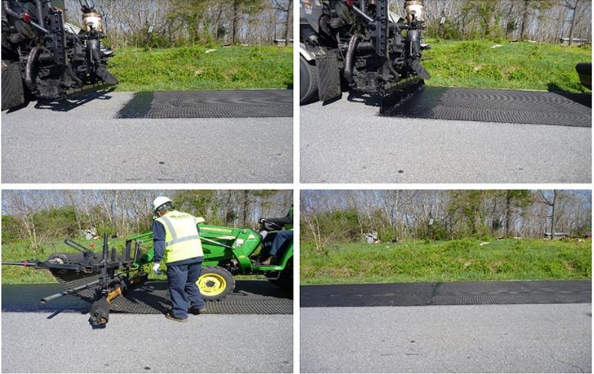
Figure 3. Longitudinal Interlayer Overlap (Route 611)
