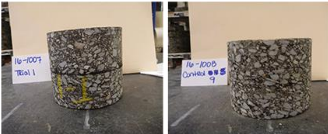
Figure 13. Cores from Route 611 Project: (left) from interlayer section; (right) from control section
