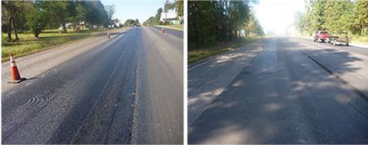
Figure 10. Emulsion Application and Overlay on US 460
