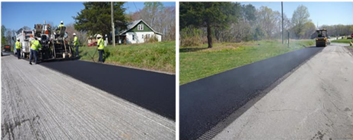
Figure 4. Asphalt Overlay Placement
