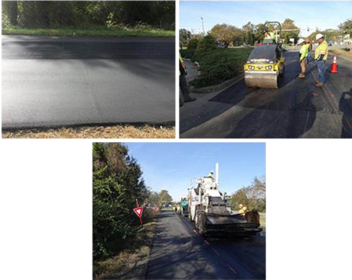
Figure 11. Interlayer and Overlay Placement on SR 30
