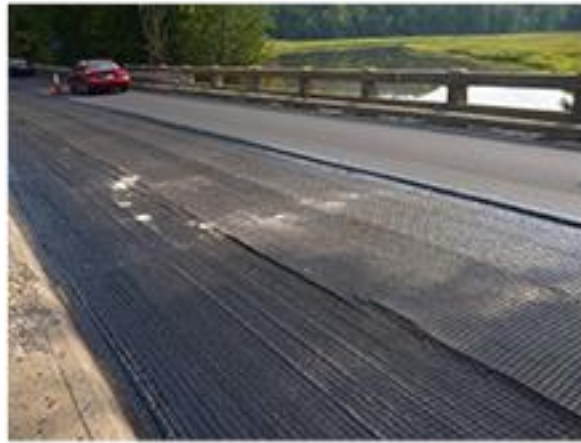
Figure 6. Fabric Placement on Route 143
