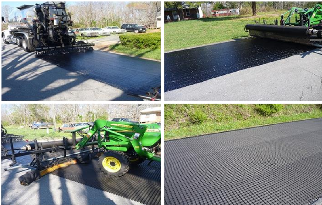
Figure 2. Interlayer Placement on Route 611
