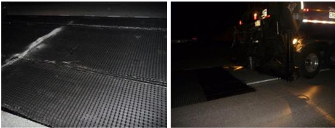
Figure 7. Fabric Placement on US 17
