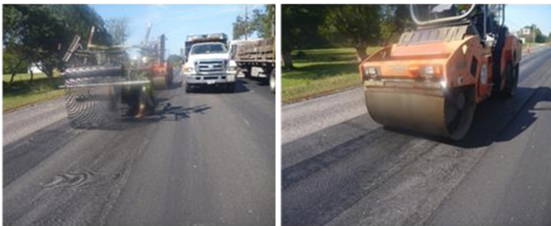
Figure 9. Interlayer Placement on US 460
