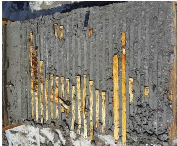
Figure 34. Result of Removal of Textured Plywood Form for Rectangular Grooves
