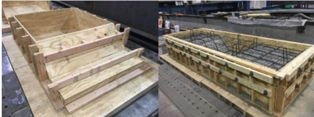
Figure 22. Sub-Assembly Formwork for Inverted T-beam (left) and CIP Topping (right)
