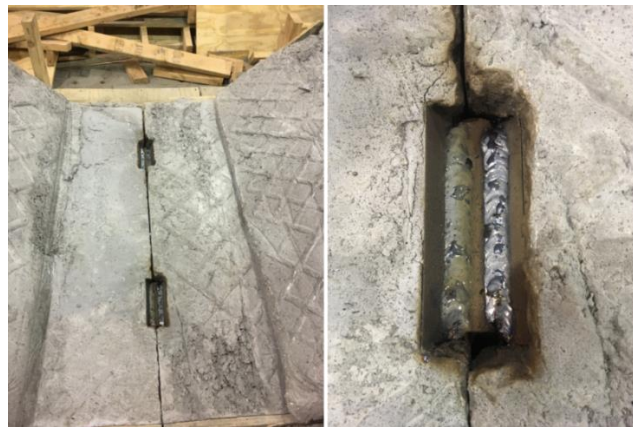
Figure 23. Welded Connection after Welding Was Completed
