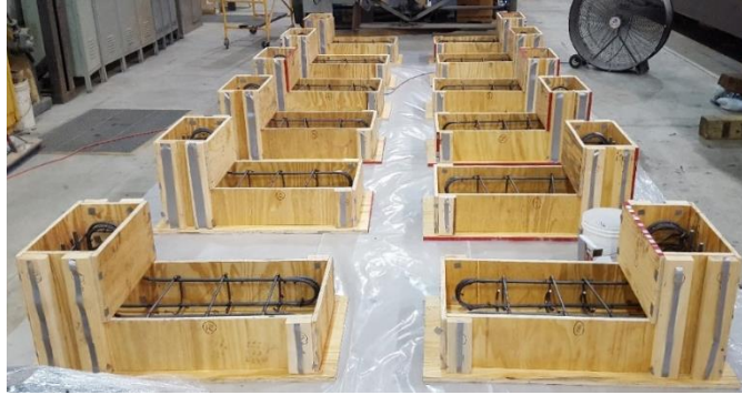
Figure 10. Forms and Reinforcing for Push-off Specimens for Bottom Section
