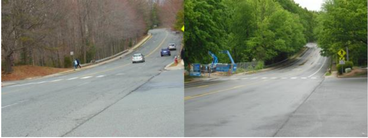
Figure 6. Before (Left) and After (Right) Photographs of Road Diet on Colts Neck Road, Southern Segment
