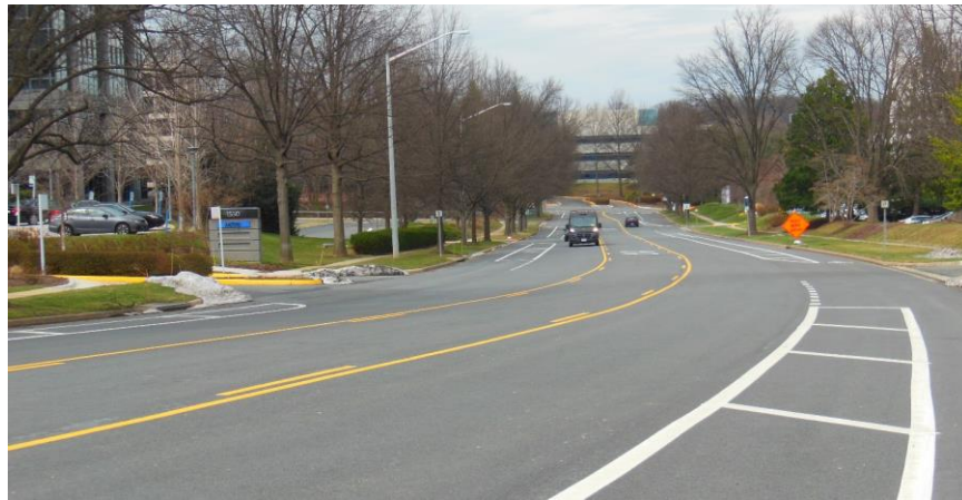
Figure 2. After Photograph of a 2016 Road Diet With Buffered Bike Lanes in Fairfax County, Virginia
