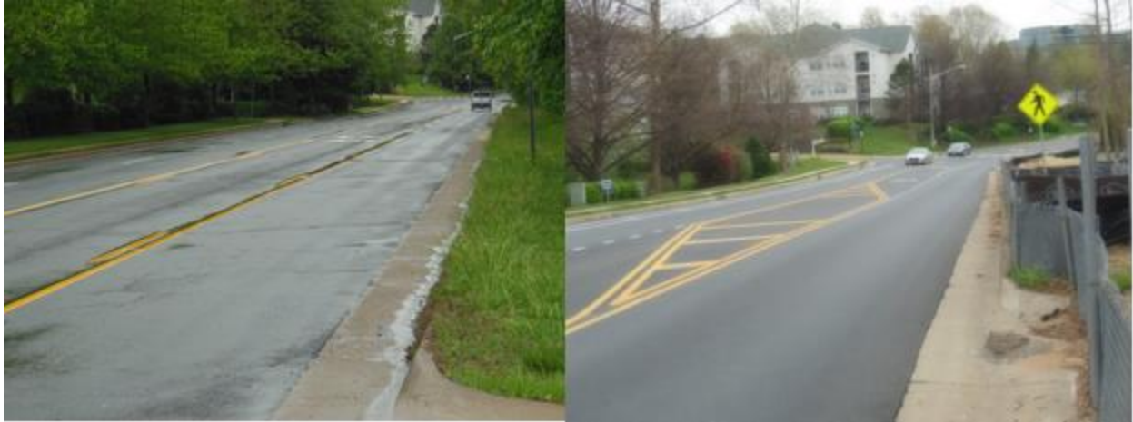
Figure 8. Before (Left) and After (Right) Photographs of Road Diet on Post Forest Drive
