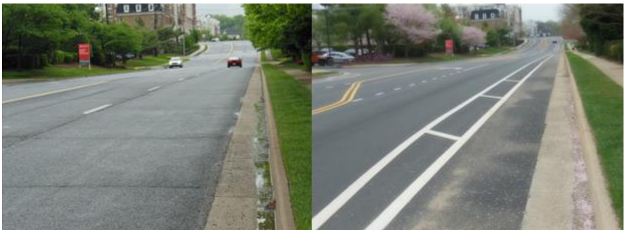
Figure 9. Before (Left) and After (Right) Photographs of Road Diet on Ridge Top Road Between Random Hills Road and Government Center Parkway
