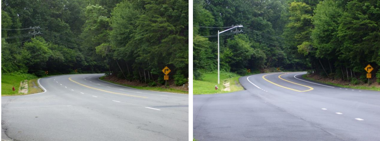
Figure 1. Before (Left) and After (Right) Photographs of a 2009 Road Diet in Fairfax County, Virginia
