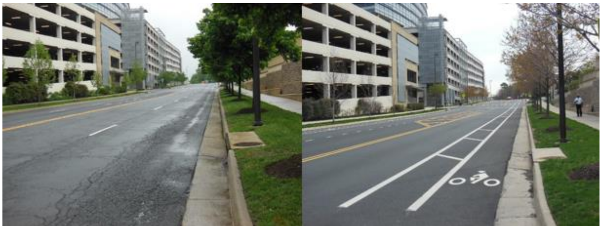
Figure 5. Before (Left) and After (Right) Photographs of Road Diet on Bluemont Way
