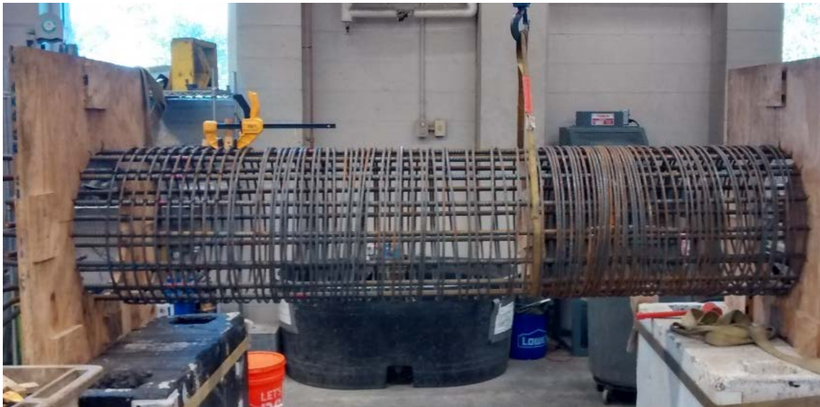
Figure 3-3. Tying column cage
