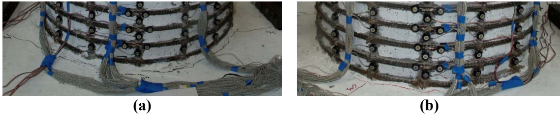
Figure 4-72. Footing Cracking: (a) F'_y on South; (b) \frac{3}{4} F'_y on North
