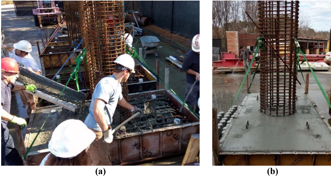
Figure 3-6. (a) Pouring footing concrete; (b) Footing concrete setting
