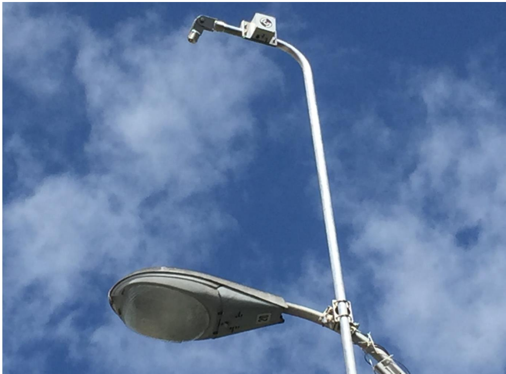
Figure 4-3. Adding Extension Structure to Increase Camera Height
