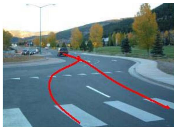
Figure 1.4 Insufficient entry path (Source: Safety Auditing Roundabouts 2004)
