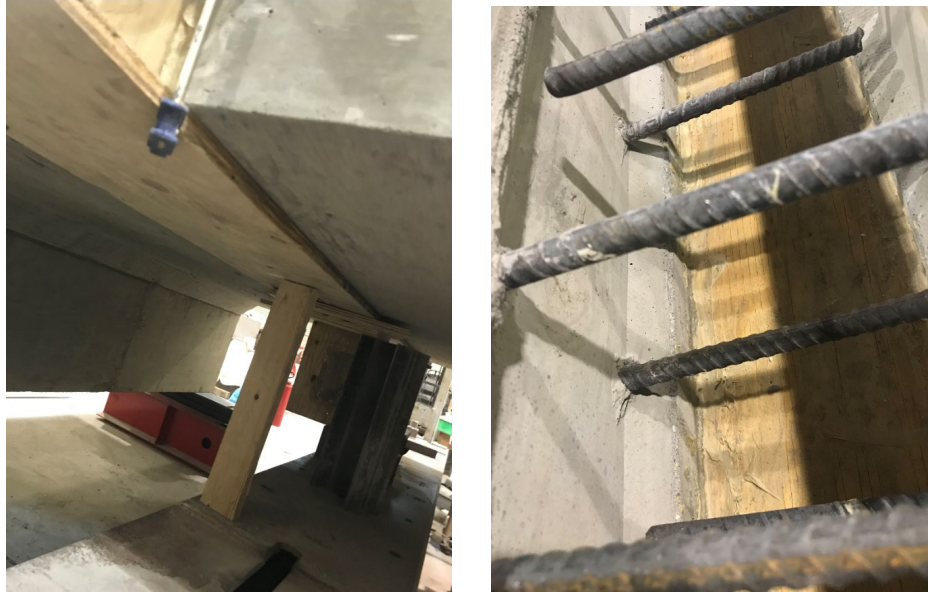
Figure 6.2 Field-scale connection formwork setup
