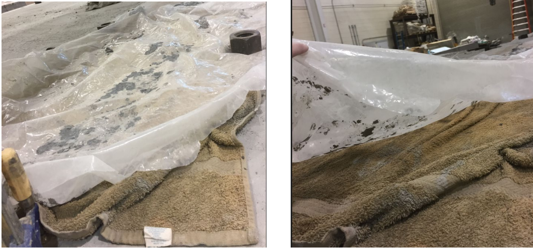
Figure 6.7 Field-scale connection UHPC curing
