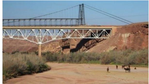
Figure 4: The U.S. 89 Bridge in Cameron, Arizona. (Image courtesy of Arizona Department of Transportation)
