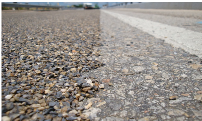
Figure 3. Photograph. Close-up view of HFST after installation.
