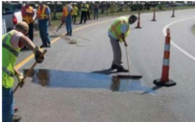
Figure 1. Photograph. HFST installation.
