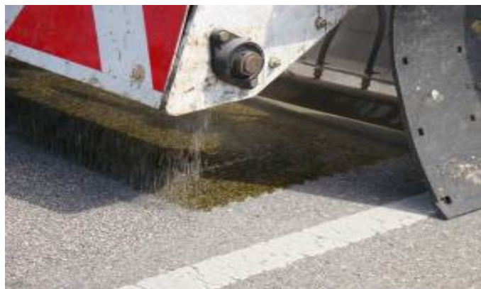
Figure 1. Photograph. HFST installation.
