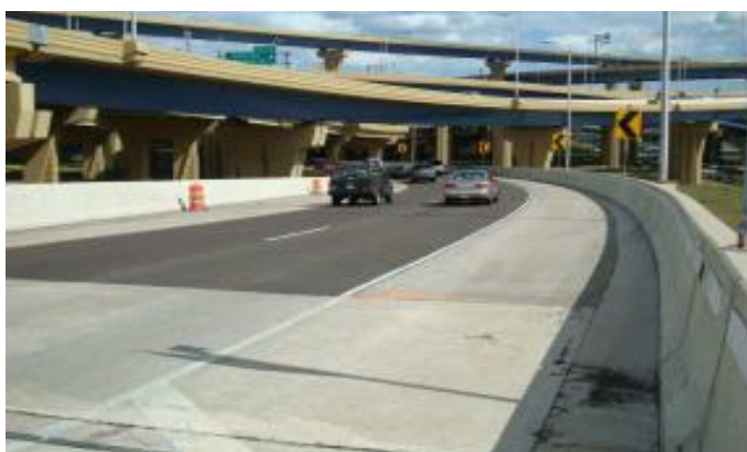
Figure 3. Photograph. Close-up view of HFST after installation.
