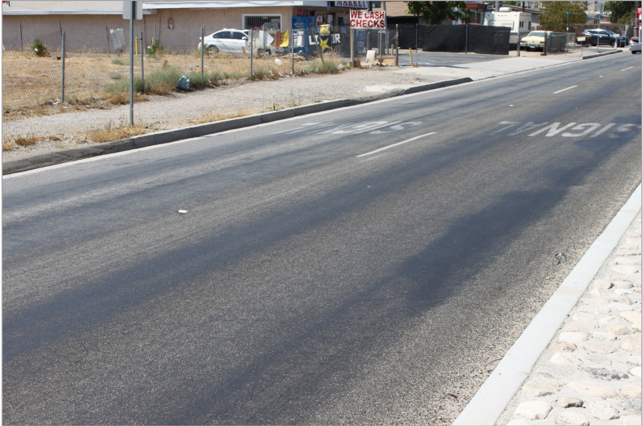
Figure 16. Photo. Rutting and wheelpath bleeding in advance of an intersection on Cedar Avenue.
