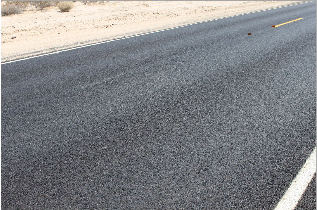
Figure 12. Photo. Scrub and fog seals applied on Silver Valley Road.
