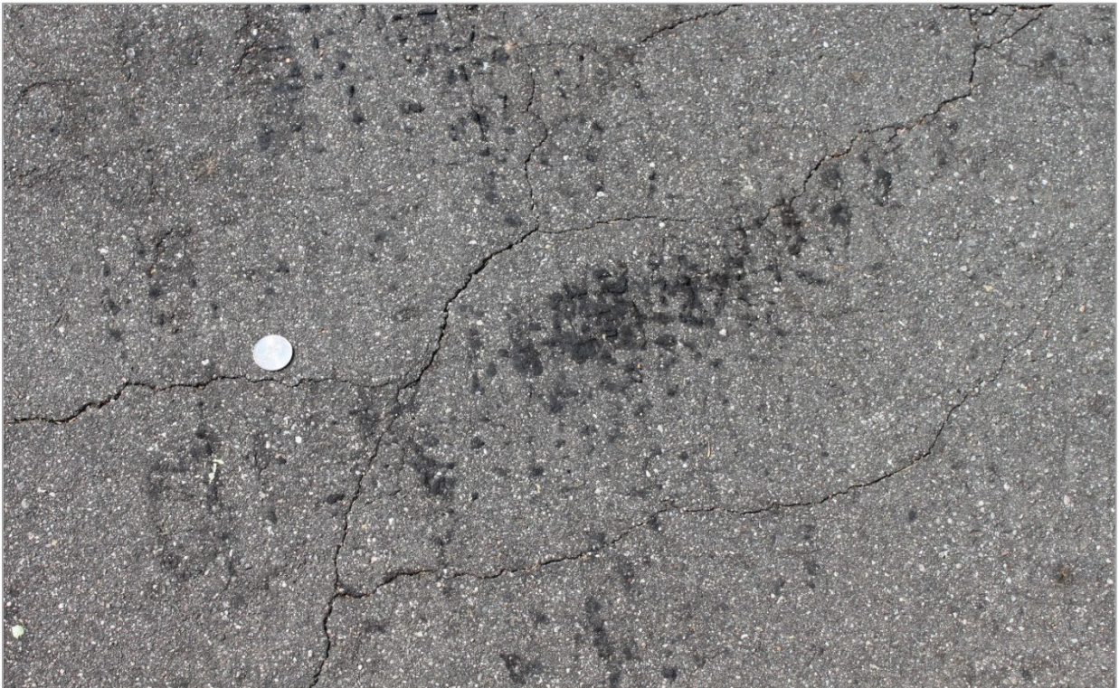
Figure 9. Photo. Four-year-old slurry seal with minor bleeding.
