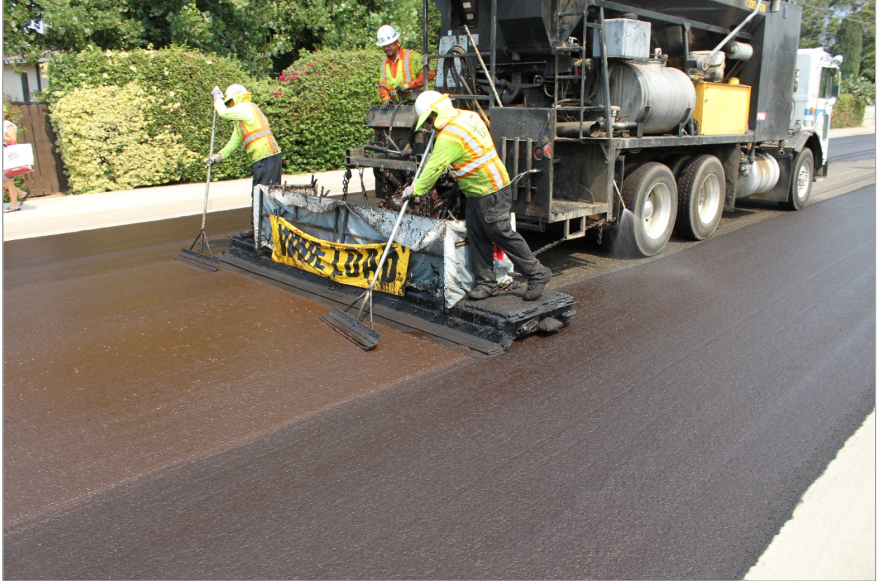
Figure 4. Photo. RAP slurry seal applied on a residential roadway in LAC.
