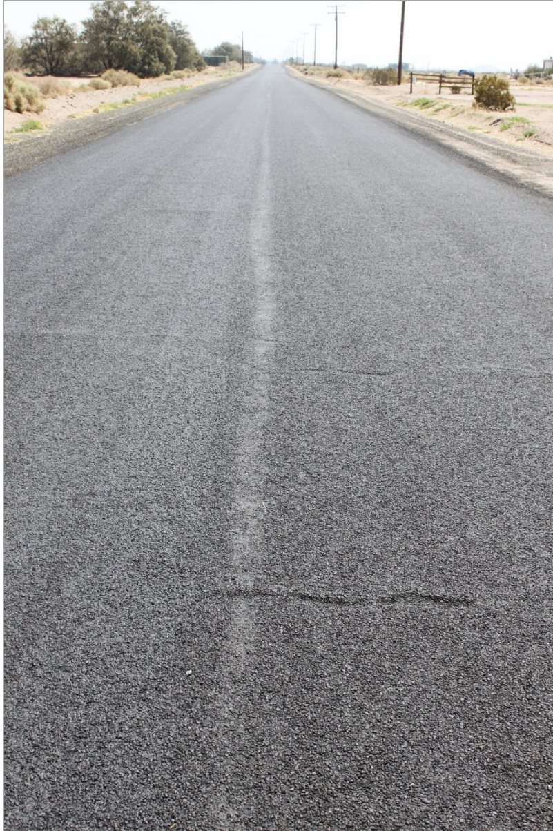
Figure 15. Photo. “Cupping” at the crack edge underneath a RAP chip seal.
