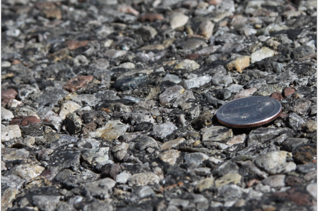
Figure 24. Photo. RAP chip seal on NM 197 with asphalt coating loss.
