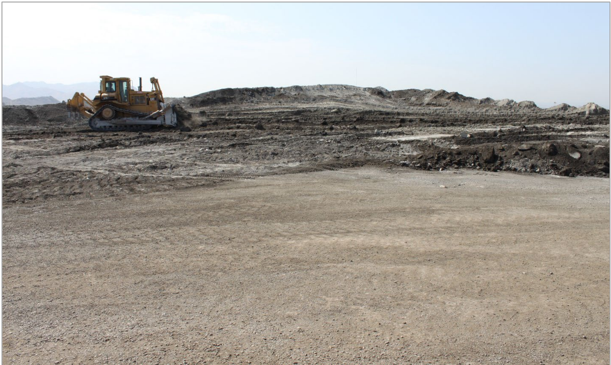
Figure 41. Photo. RAP excavation from a stockpile for processing into chip and fine fractions.
