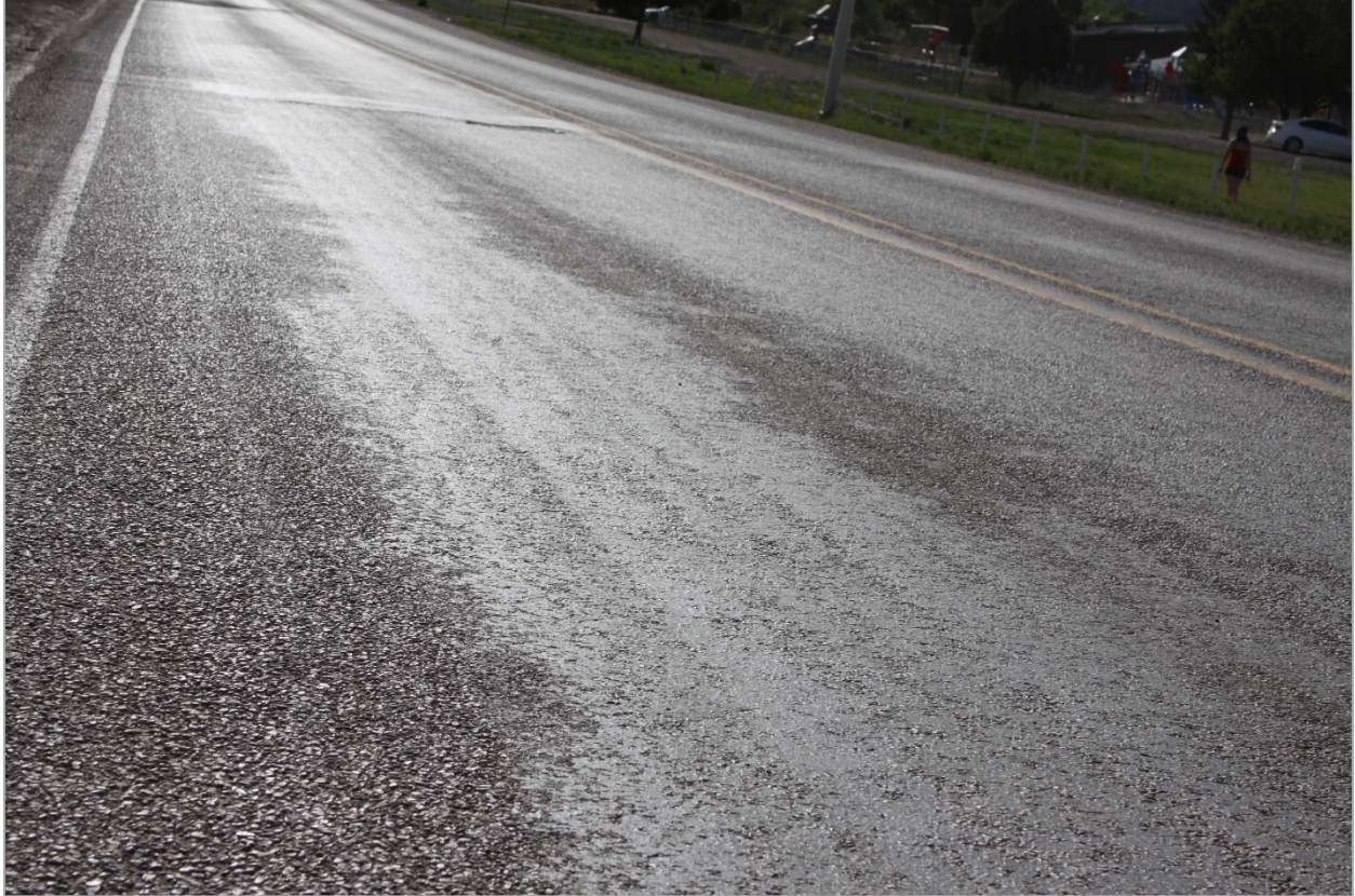
Figure 23. Photo. RAP chip seal on NM 126 with flushed wheelpaths.
