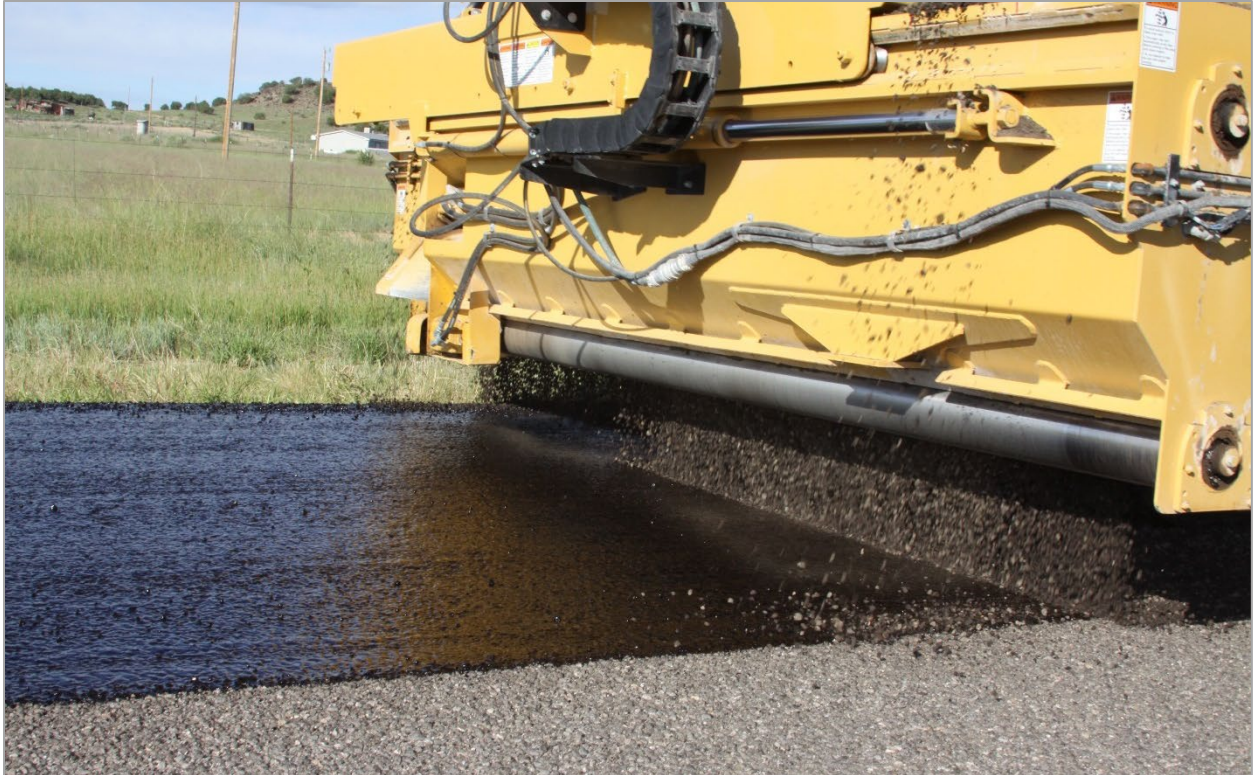
Figure 21. Photo. Chip spreader applying RAP chips on NM 126 (Tarefder and Ahmad 2017).
