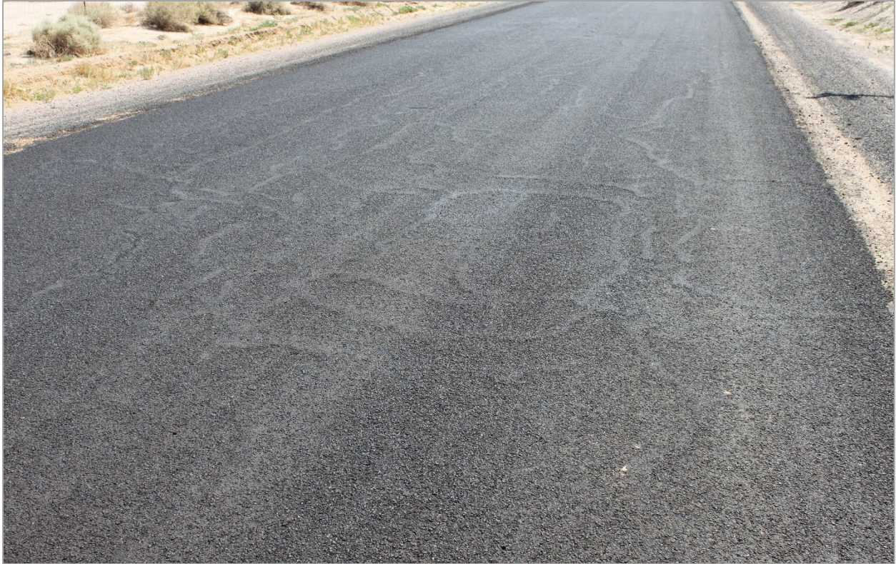
Figure 14. Photo. RAP chip seal applied over extensive crack filling.
