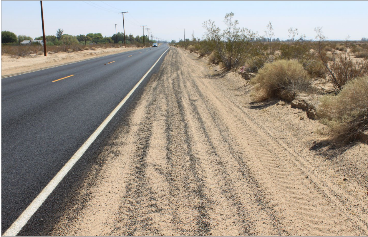
Figure 13. Photo. Minimal chip loss on Mineola Road.
