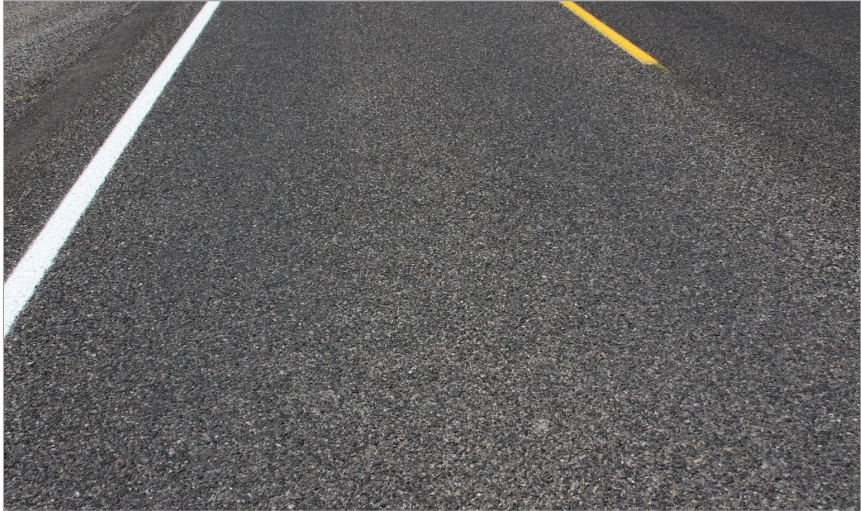
Figure 22. Photo. RAP chip seal applied on NM 124.
