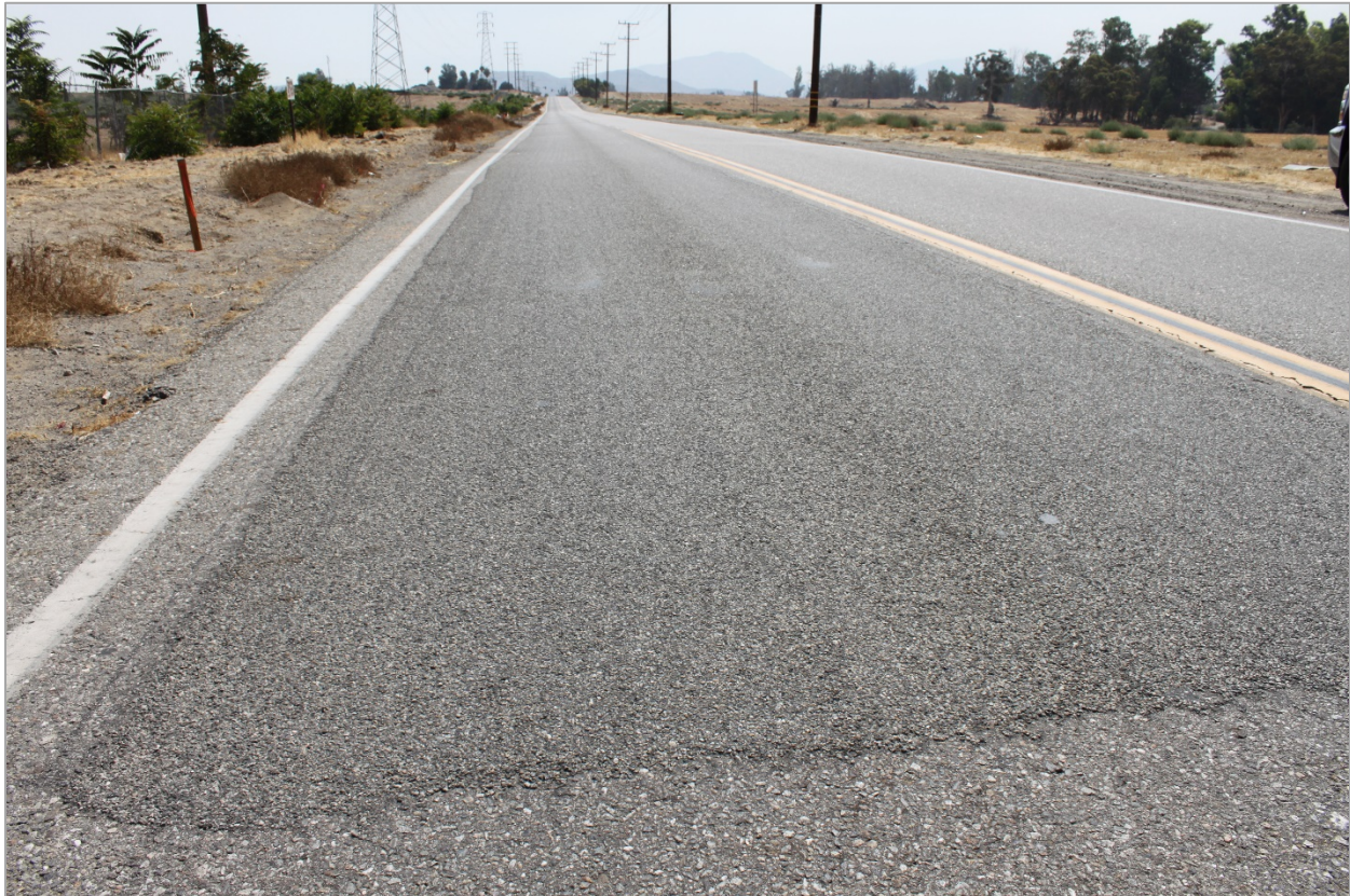
Figure 43. Photo. PPTA’s first RAP chip seal test section.
