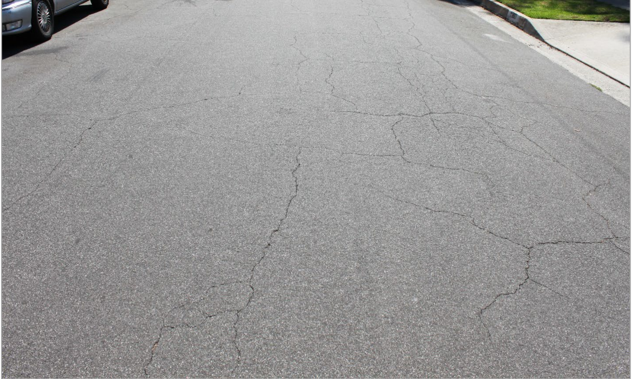
Figure 8. Photo. Four-year-old slurry seal with low-severity block cracking.
