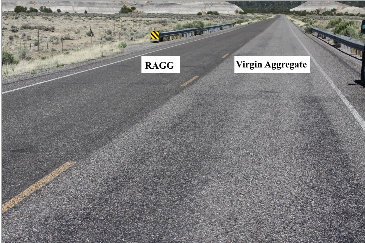
Figure 26. Photo. Color difference between a surface treatment using RAGG and another using virgin aggregate on NM 197.
