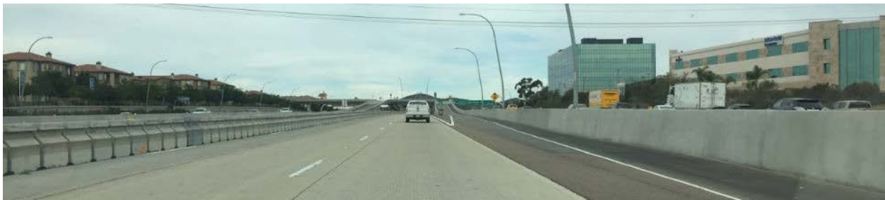
Fig 21. Movable Barriers along I-15 Express Lane (on left side).
