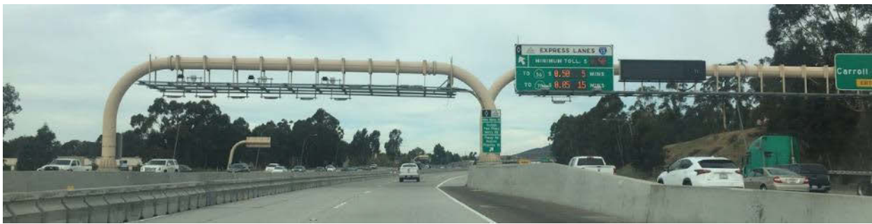
Fig 23. Changeable Message Signs on I-15 Express Lane.
