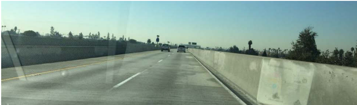
Fig 14. Elevated Express Lane Facility on I-110.
