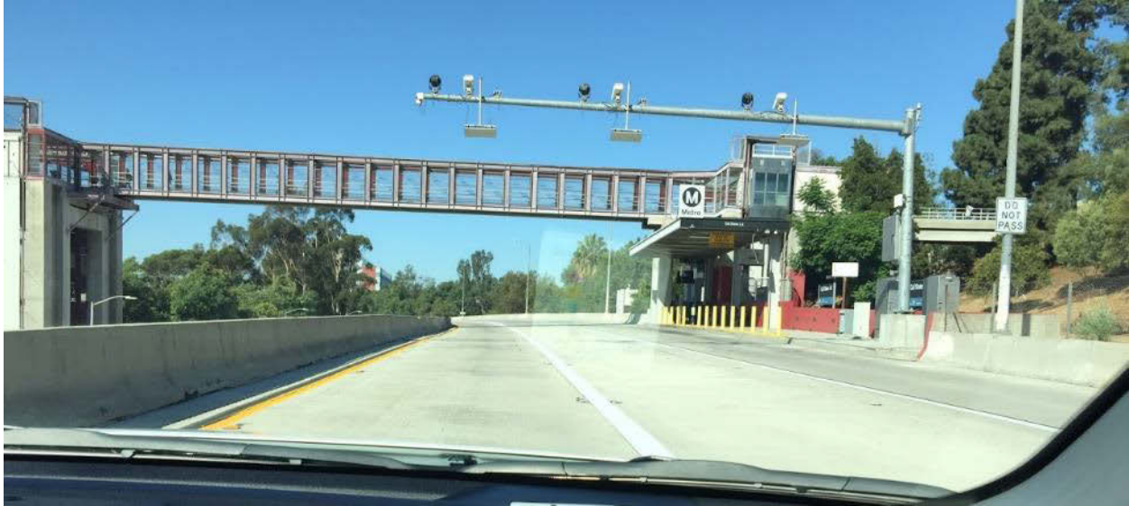
Fig 12. Bus Station at the I-10 Express Lane Facility.
