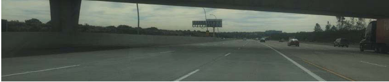
Fig 22. Permanent Barriers along I-15 Express Lane.
