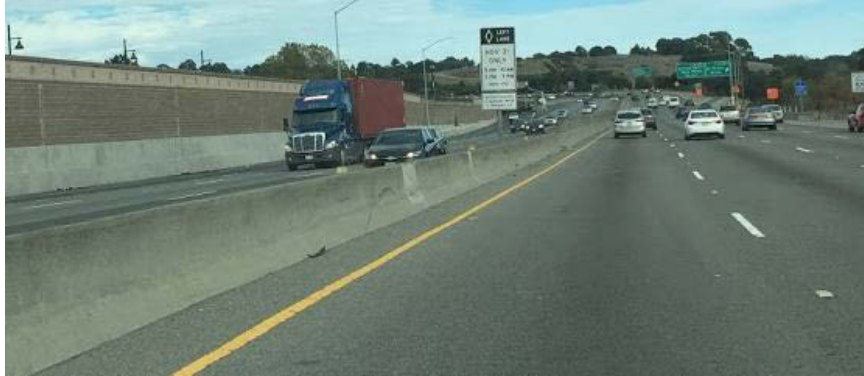
Fig 2. Left Shoulder of the I-80 HOV Lane.
