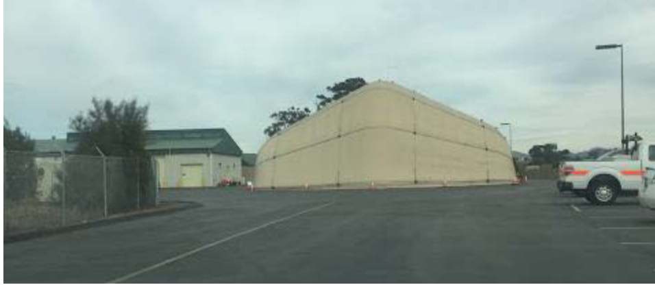
Fig 24. South Control Yard on the Southern End of I-15 Express Lane.
