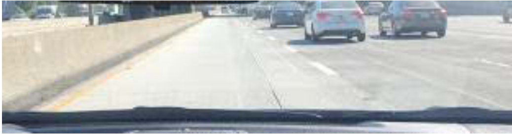
Fig 8. No Left Shoulder along the I-210 HOV Lane.
