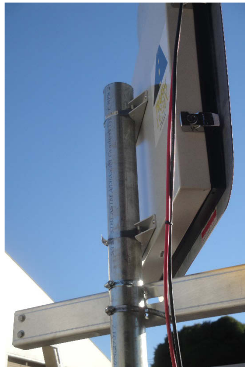
Figure 4.6 VSA sign and solar panel wire connection
