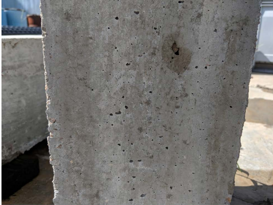
(a) Cracking Index - 0.01 in/yd (Visual Rating – 1.5)
