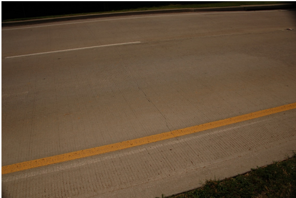
Figure 3.9: Northbound frontage road
