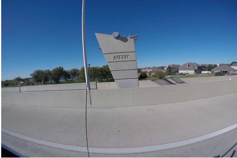
Figure 3.20: Southbound main lane. Pavement in excellent condition as recorded by video
