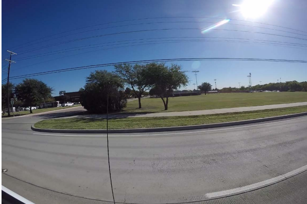
Figure 3.18: Northbound frontage road. Pavement in excellent condition as recorded by video
