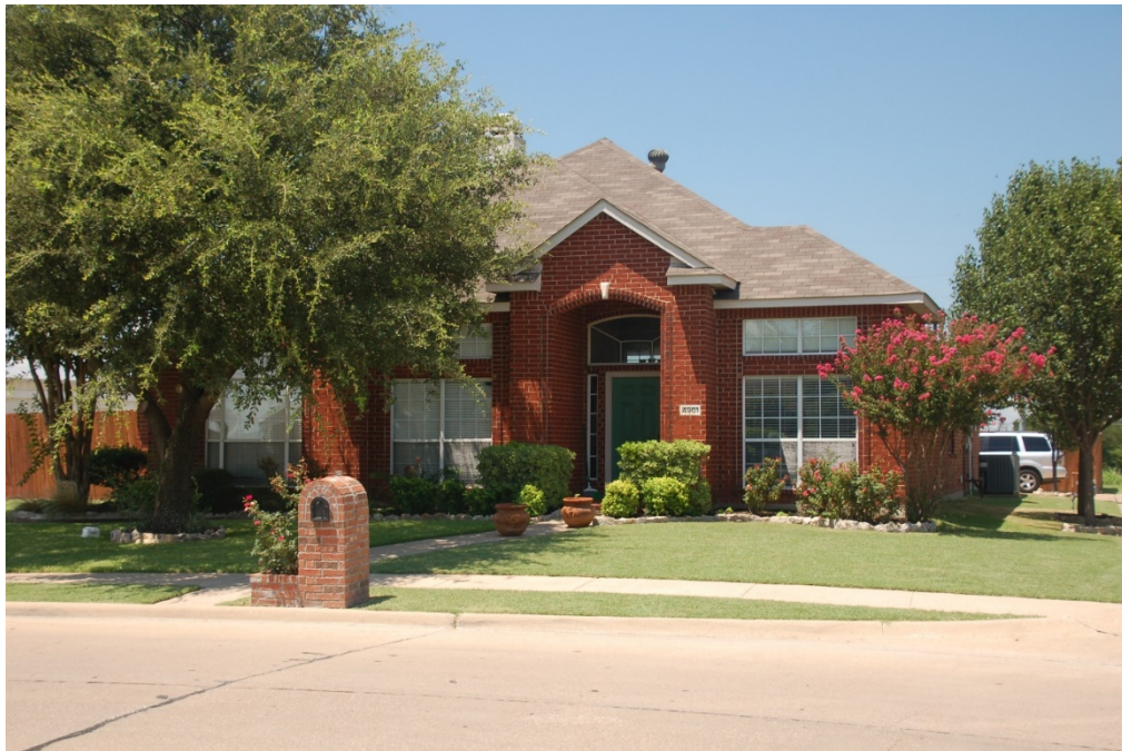
Figure 2.12: Front view of Site #3: 4901 Harborview Dr.
