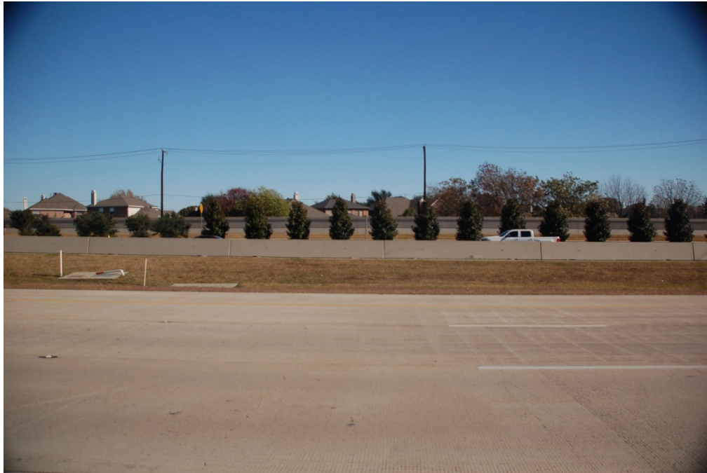
Figure 3.5: Southbound main lanes
