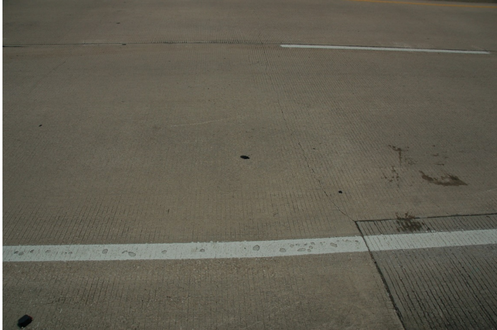
Figure 3.6: Northbound frontage road
