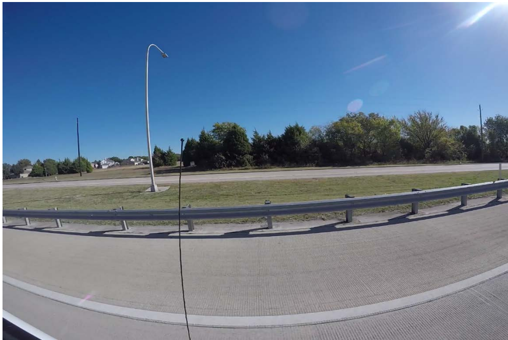
Figure 3.17: Northbound main lane. Pavement in excellent condition as recorded by video
