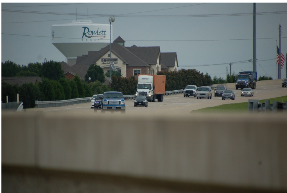
Figure 1.7: View 2 of the southbound main lanes
