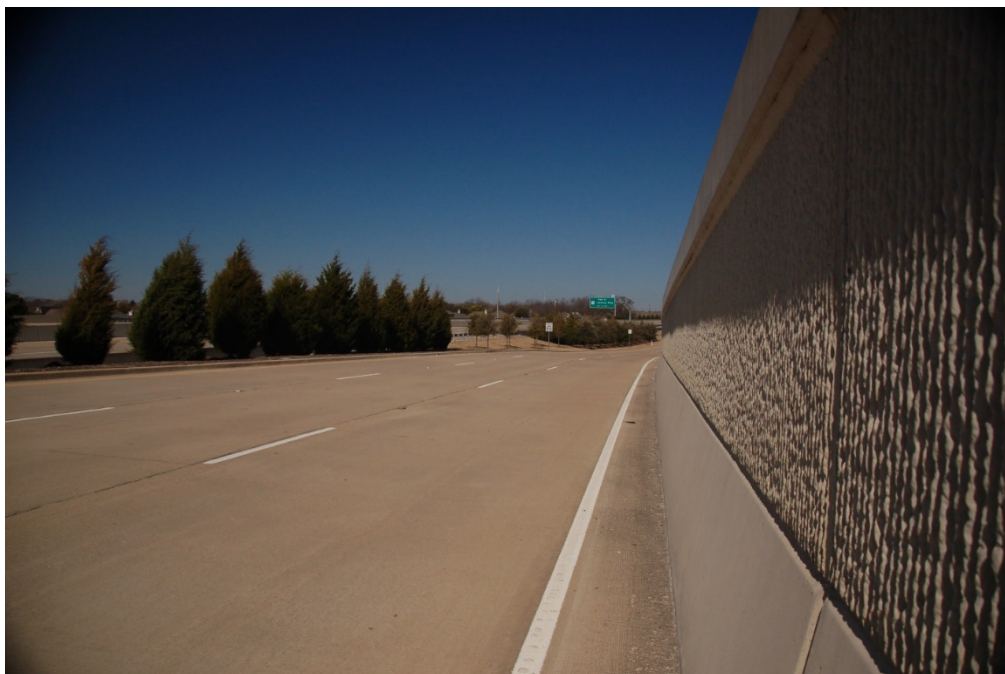
Figure 1.8: View 1 of the northbound frontage road
