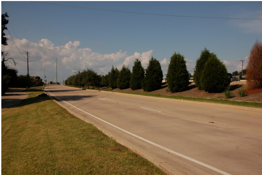
Figure 1.11: View of the southbound frontage road
