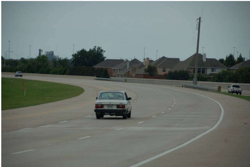
Figure 3.7: Southbound main lanes
