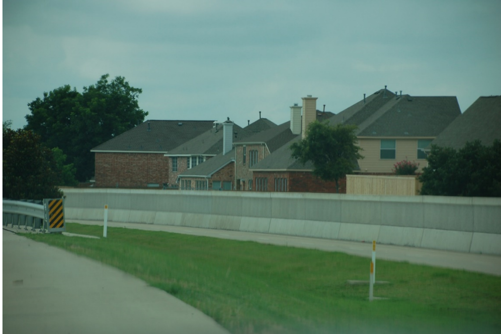
Figure 1.15: View of the west noise wall from the westbound main lanes
