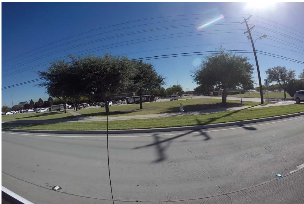
Figure 3.15: Northbound frontage road. Transverse cracks as recorded by video
