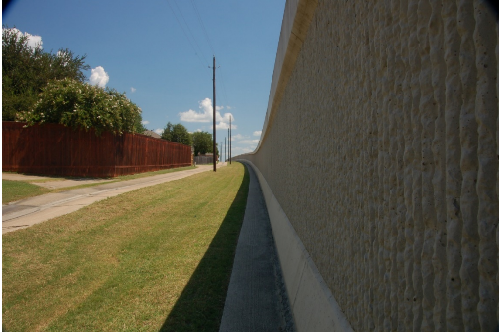
Figure 1.13: View of the east noise wall from the neighborhood side
