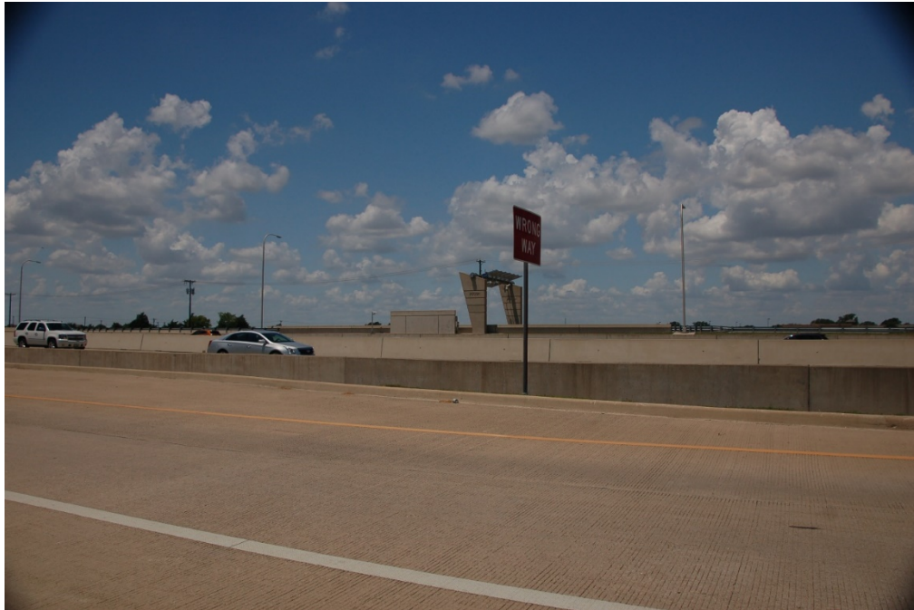
Figure 3.10: Northbound exit ramp
