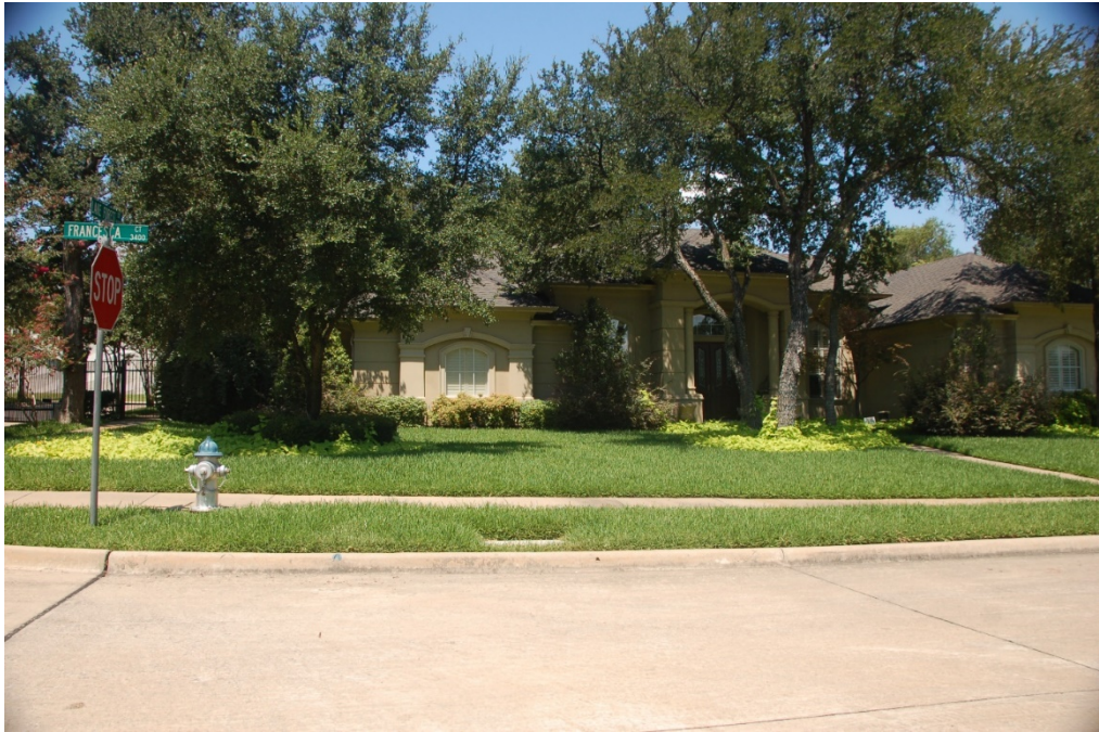
Figure 2.16: Front view of Site #4a: 3401 Francesca Ct.
