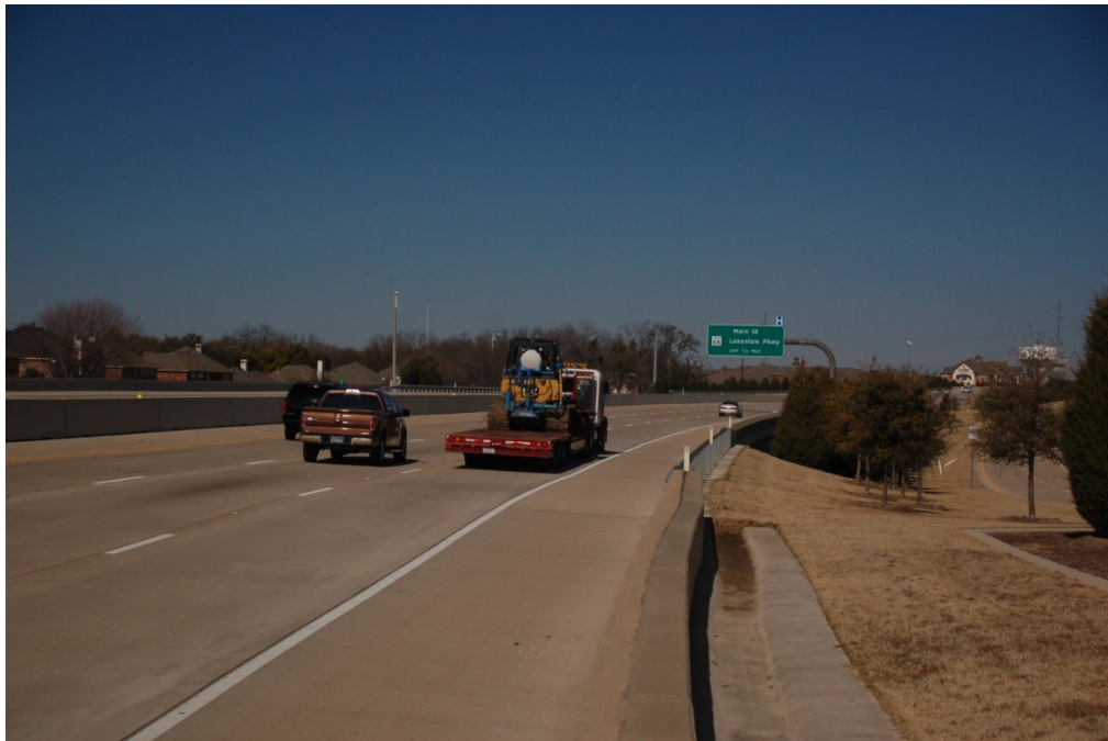
Figure 1.5: View 2 of the northbound main lanes
