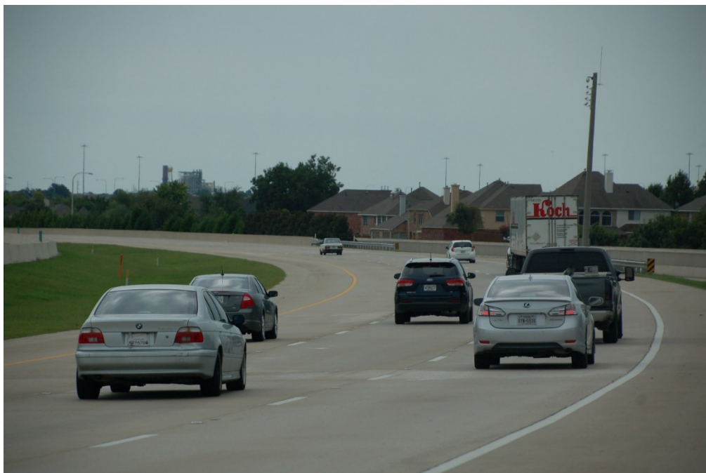
Figure 1.6: View 1 of the southbound main lanes
