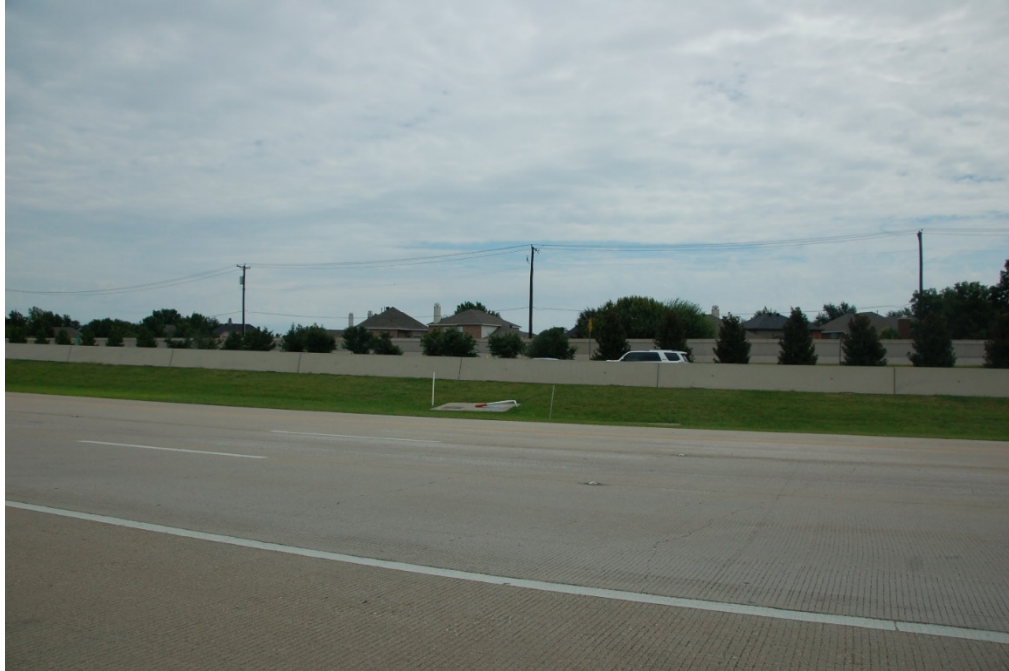
Figure 3.8: Southbound main lanes
