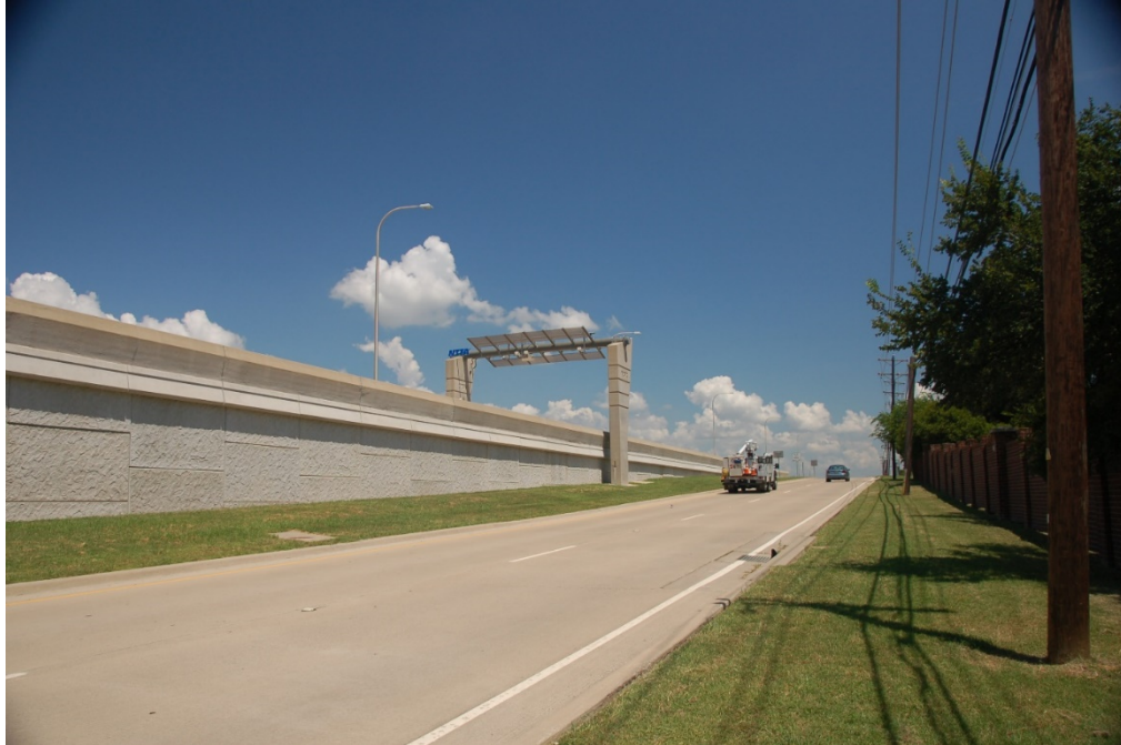
Figure 1.10: View 3 of the northbound frontage road
