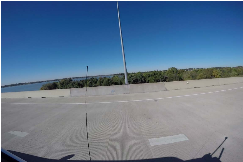
Figure 3.21: Southbound main lane. Pavement in excellent condition as recorded by video
