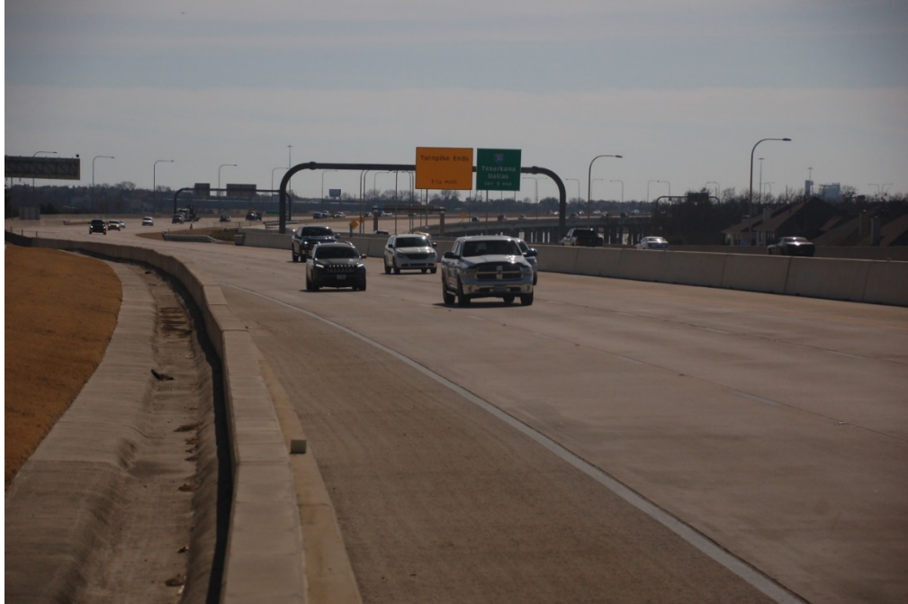
Figure 1.4: View 1 of the northbound main lanes
