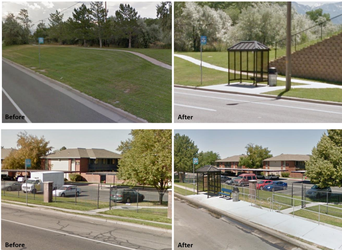
Figure 3.2. Before and after bus stop facility improvements along the #41 bus line.
