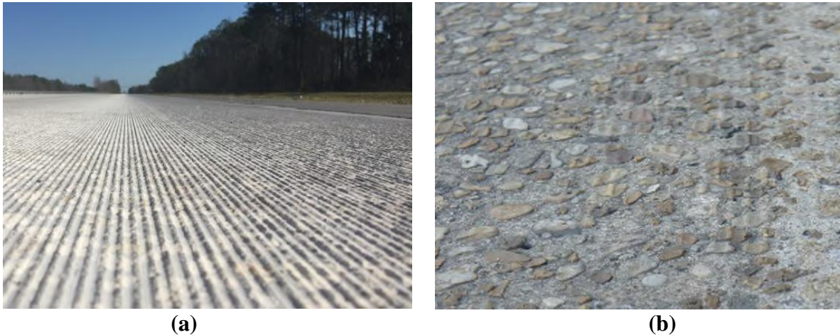
Figure 18. (a) New and (b) old longitudinally-ground surfaces (after Holzschuher, 2017a)
