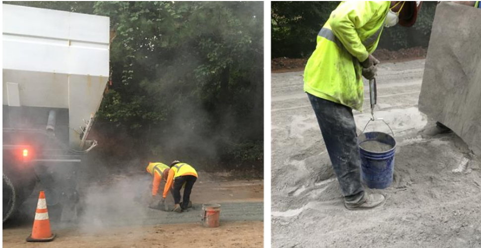
Figure 6. Photos. Dry cement placement and cement spread rate check.
