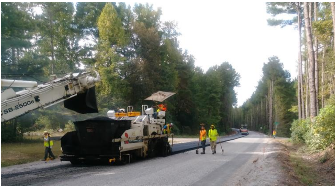
Figure 13. Photos. Asphalt concrete surface placement (10/3/2018).
