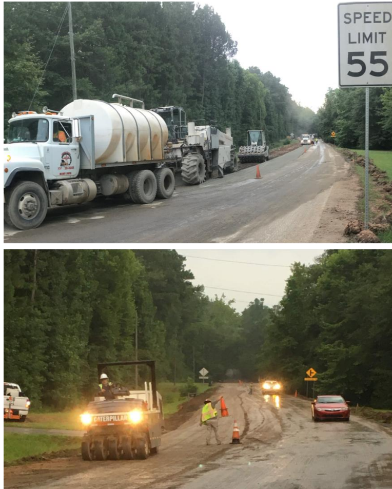
Figure 7. Photos. Pulverization and compaction of the FDR base.
