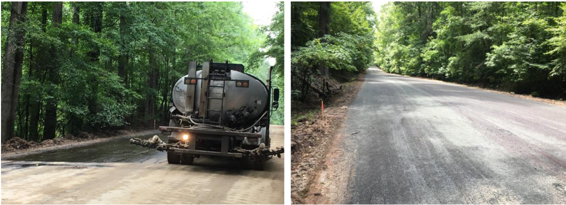
Figure 11. Photos. Placement of the chip seal layer.
