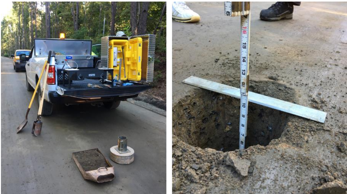
Figure 10. Photo. Density, moisture content and thickness verification (performed by GDOT).
