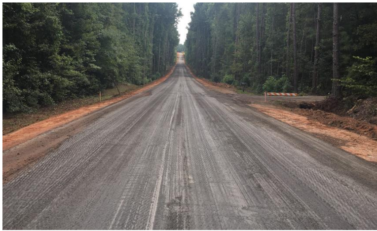
Figure 4. Photo. Asphalt milling.
