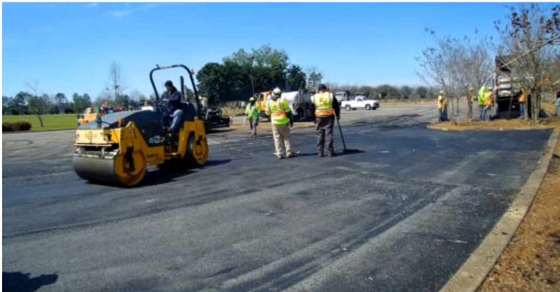
Figure 8. Photo. Jobsite scene of the preliminary test.
