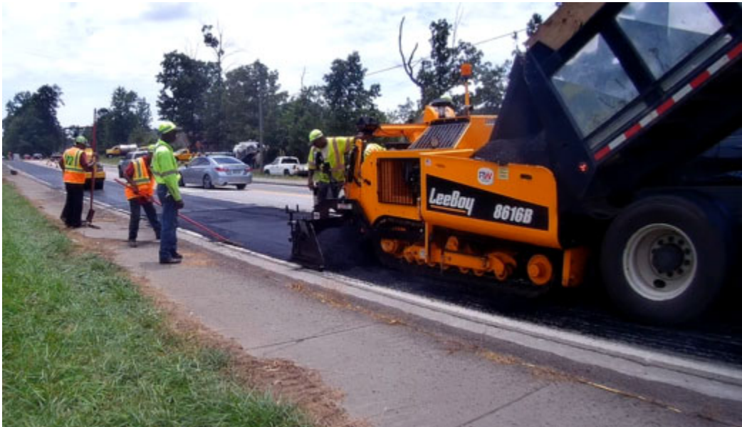
Figure 13. Photo. Jobsite scene of the first evaluation test.
