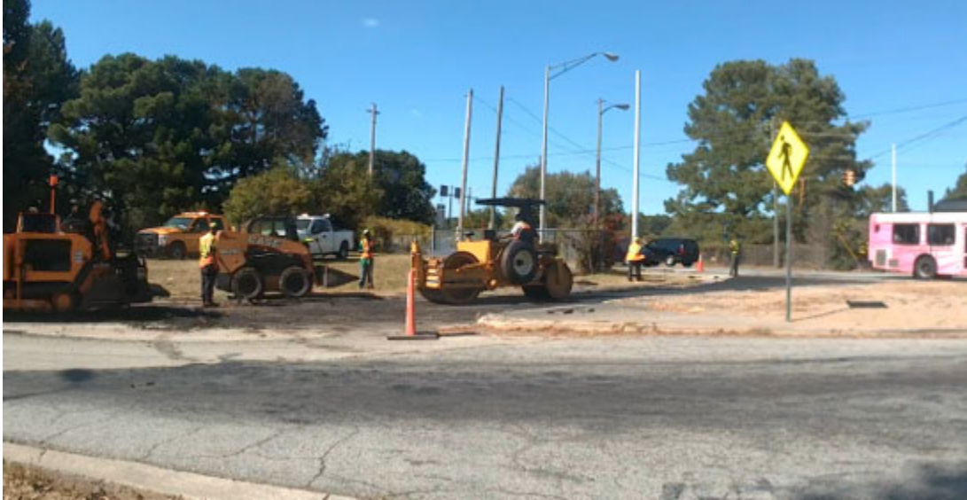
Figure 15. Photo. Jobsite scene of the third evaluation test.
