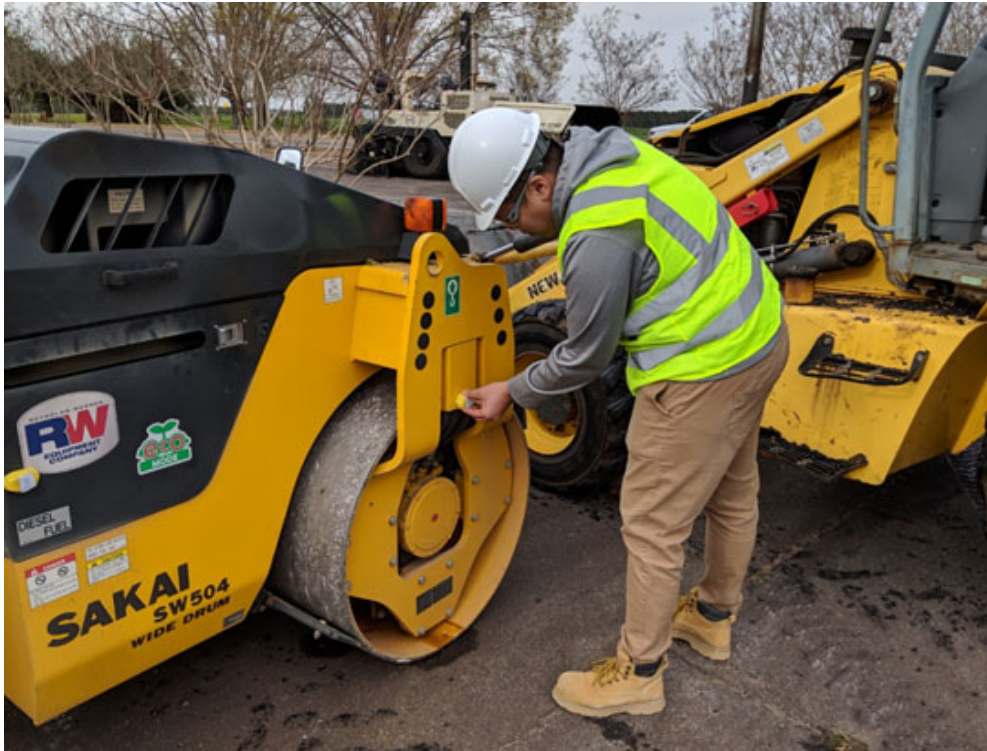
Figure 5. Photo. Sensor installation.
