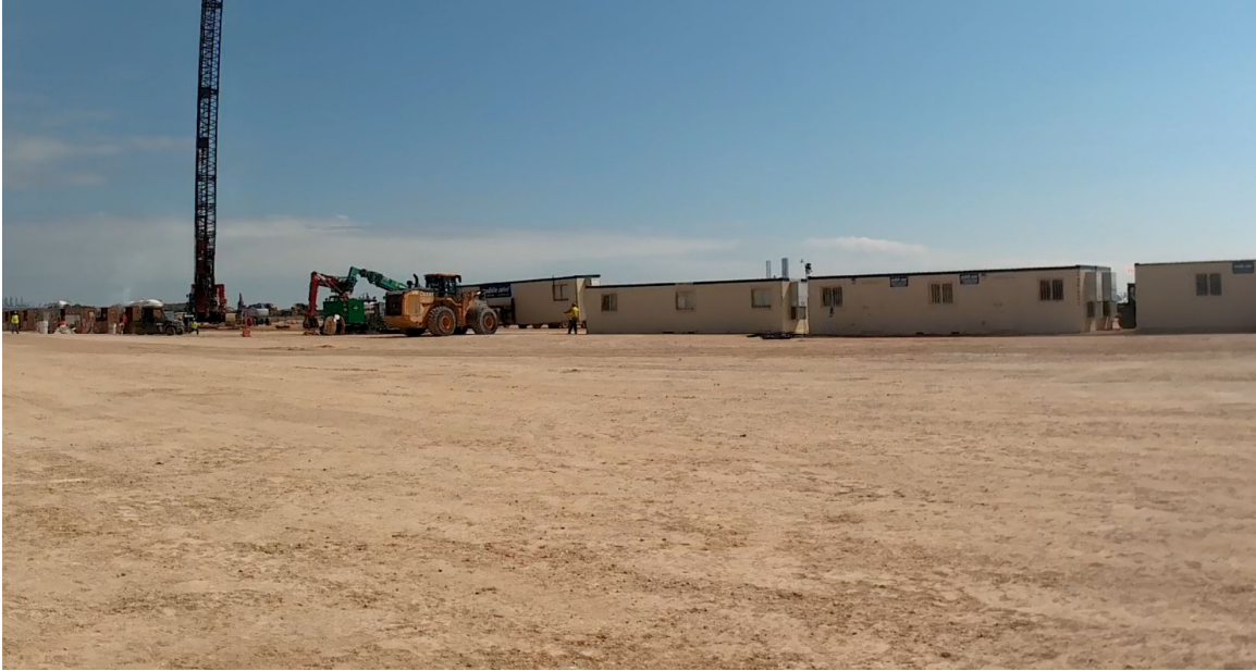
Figure 16. Photo. Jobsite scene of the fourth evaluation test (side view).
