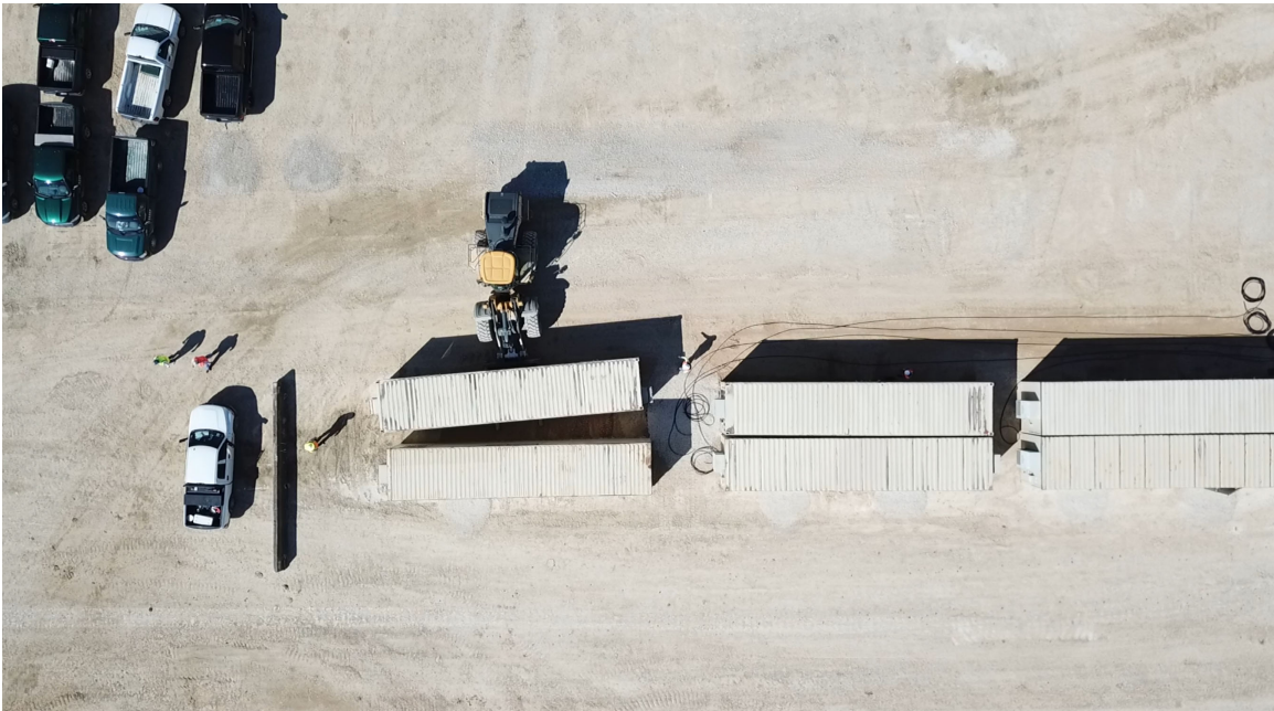
Figure 17. Photo. Jobsite scene of the fourth evaluation test (top view).
