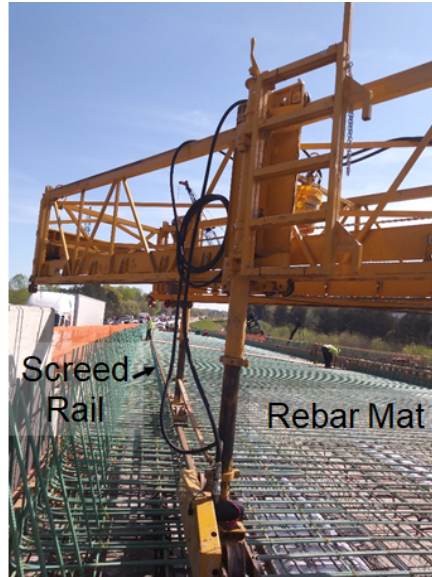
Figure 3. Photo. Key elements of the cover verification process.
