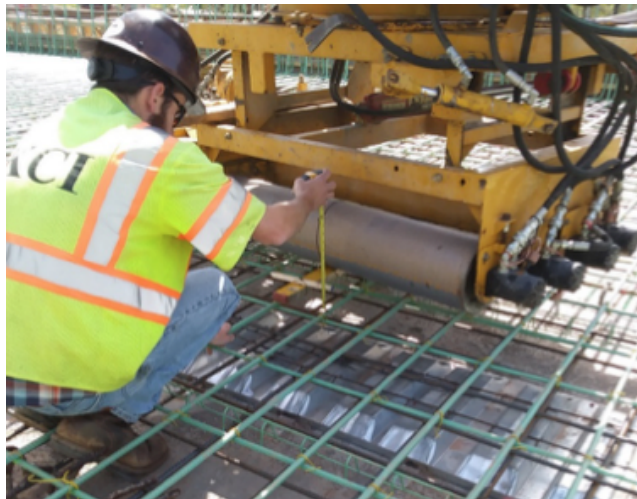
Figure 5. Photo. GDOT inspector measuring the concrete cover using a tape measure and lumber affixed to the bottom of the screed head.
