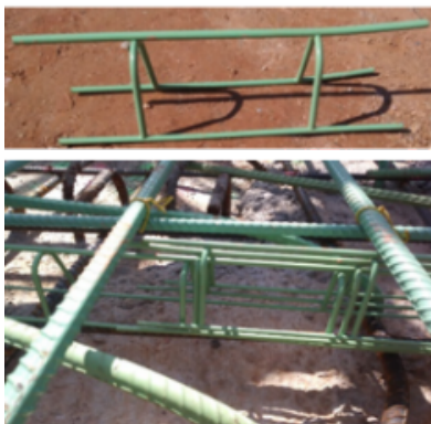
Figure 4. Photo. Chairs used to set appropriate standoff distance between rebar mats.
