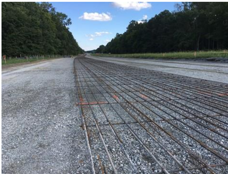
Figure 7. Reinforcement for CRCP. CRCP = continuously reinforced concrete pavement.
