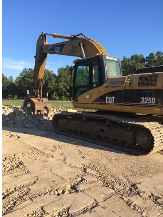
Figure 4. Crushed Concrete Being Removed
