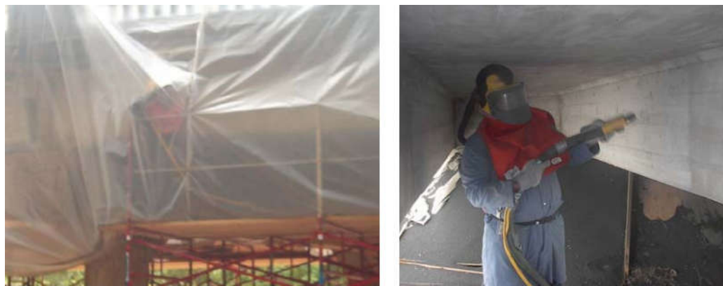
Figure 4-2. Surface Preparation by Sand Blasting
