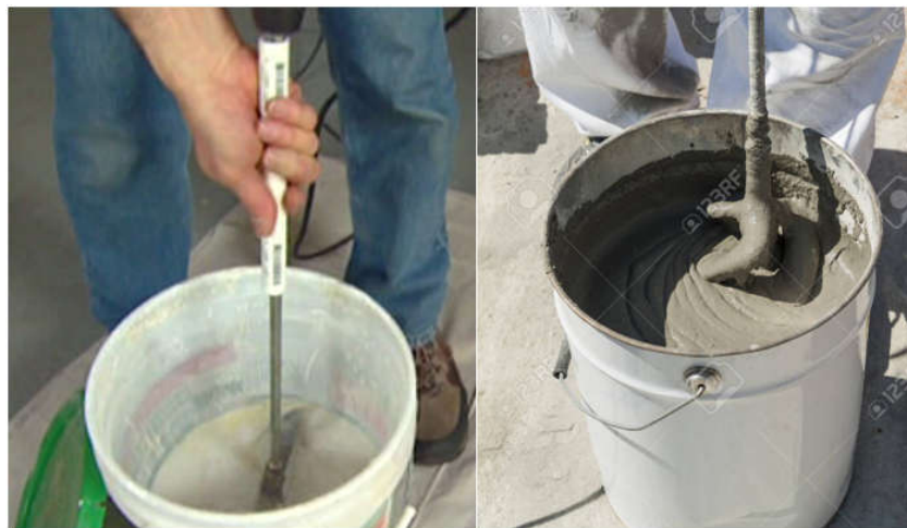
Figure 4-4. Mixing Resin and Cementitious Matrix
