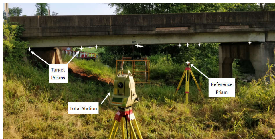
Figure 5-4. Total Station Setup
