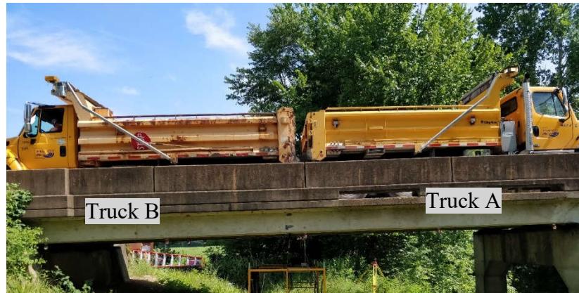
Figure 5-7. Trucks on Span 1 for Load Test
