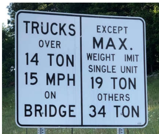
Figure 3-1. Bridge P-0058 Load Posting
