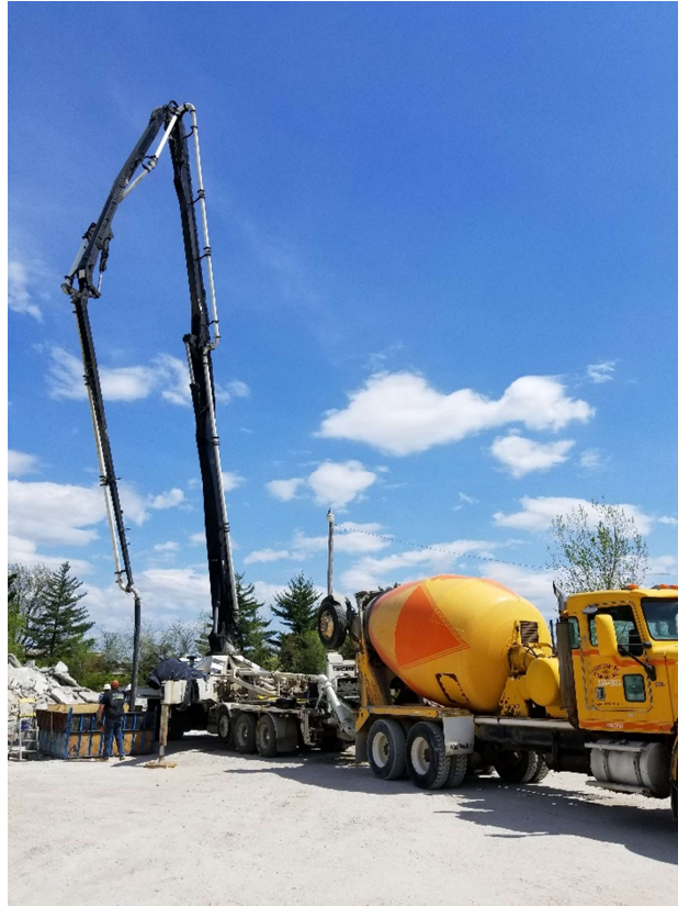
Figure 59. Pumping boom in A-shape configuration.
