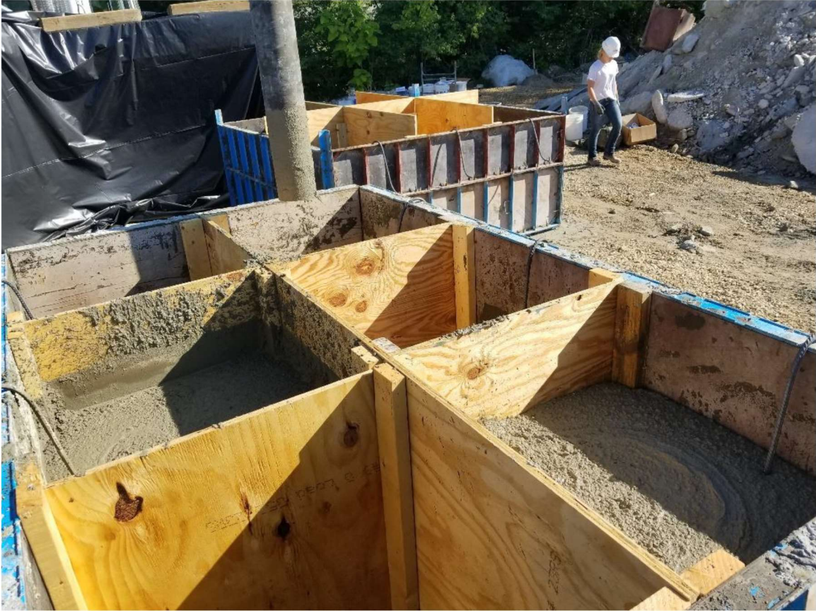
Figure 61. Formworks to hold approximately 800 l of concrete.
