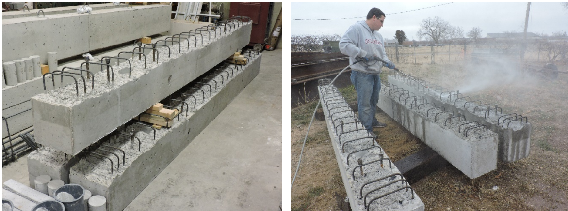
Figure 5.10: Preparation of Class AA Substrate for Full-Scale FR-SCC Repaired Beam Specimens
