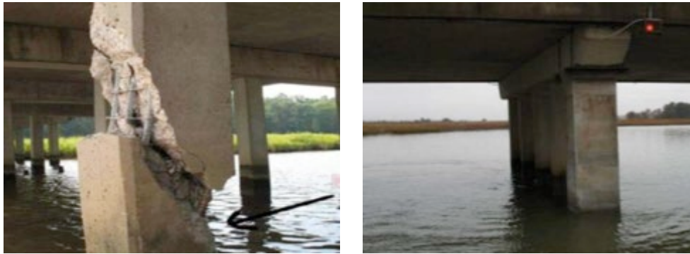
Figure 1.2: SCC Used in the Repair of Bridge Piles (Ozyildirim, 2013)
