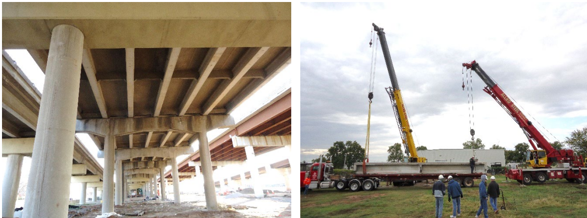
Figure 6.3: Control Girder Span Location on Bridge (l) and Delivery to Structures Lab (r)
