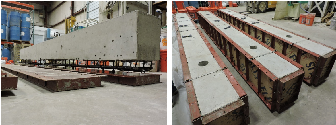
Figure 5.11: Preparation for FR-SCC Repair Material Placement
