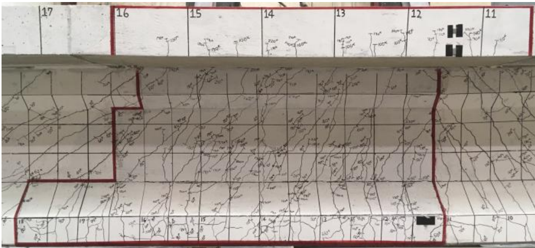
Figure 6.18: North End Region Repair at End of C2 Support Condition Testing
