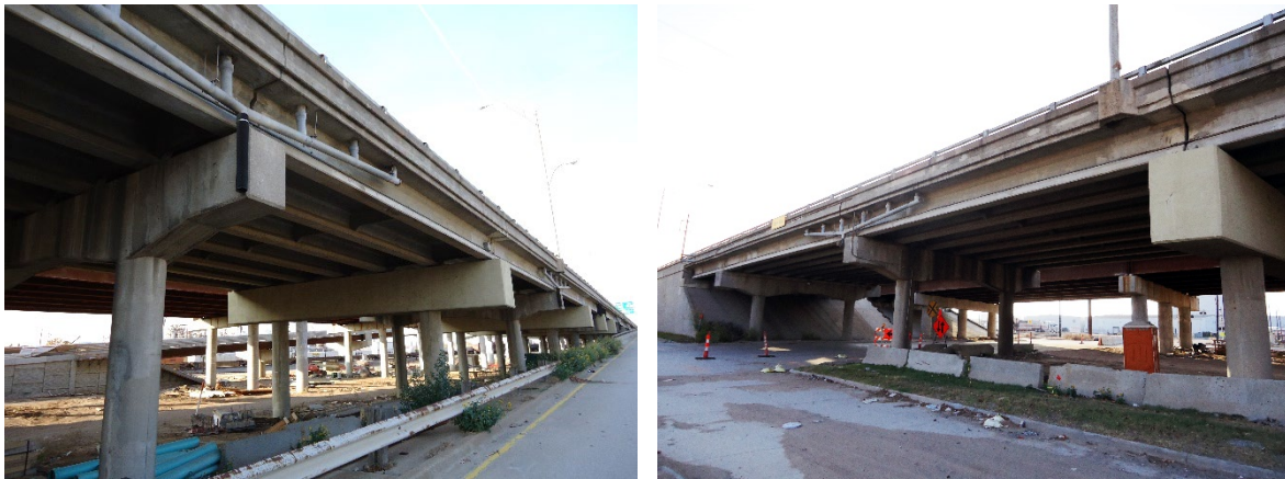
Figure 6.1: Overall Views of the I-244 Bridge Over the Arkansas River
