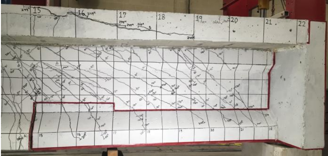
Figure 6.17: South End Region Repair at End of C1 Support Condition Testing
