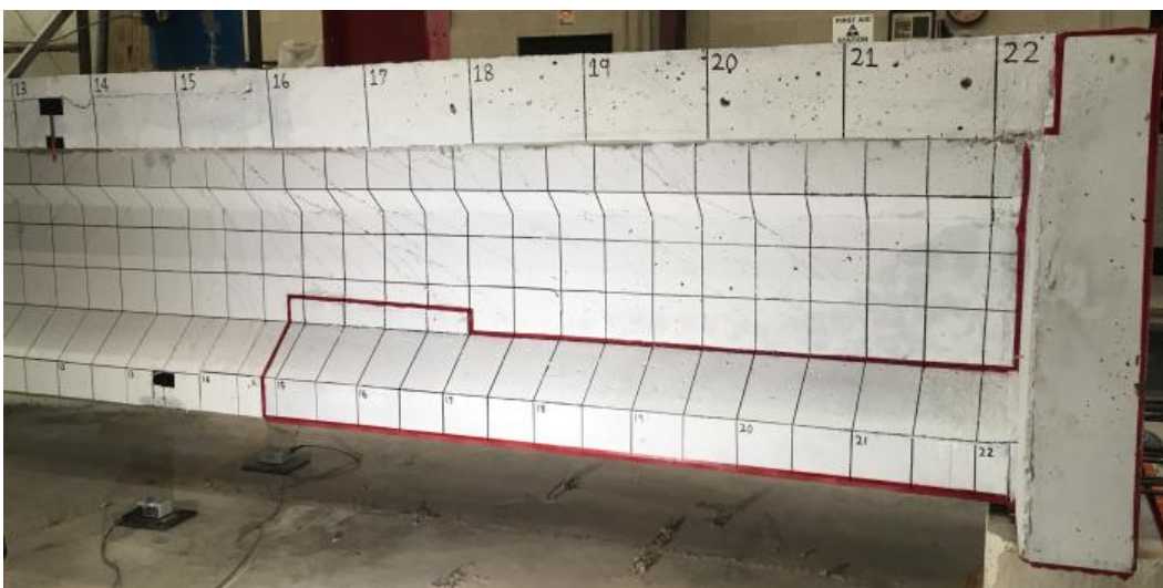
Figure 6.13: Photograph of Girder South End FR-SCC Repaired Region
