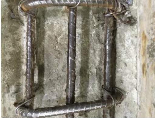
(a) Cleaned reinforcement before repair
