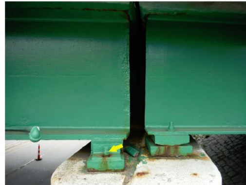
Photo 11: Heavy section loss to the anchor bolt nut of the Beam 37 bearing at Pier 2 in Span 5.
