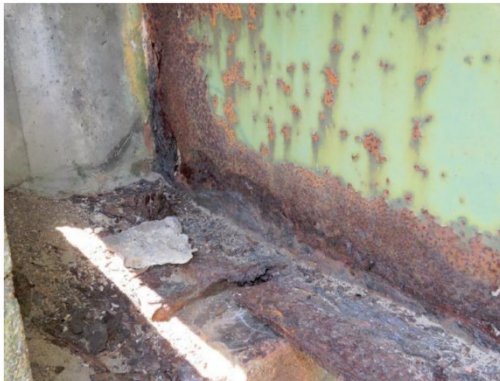
Photo 9: Beam #6 at the South end.
