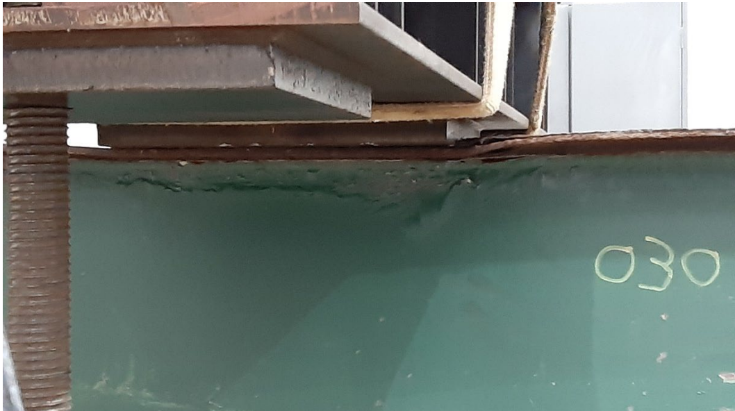
Figure 6.34: Web crippling observed underneath area of loading.
