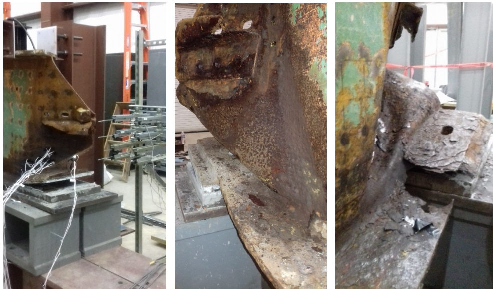
Figure 6.12: Residual deformation after unloading Specimen 2.
