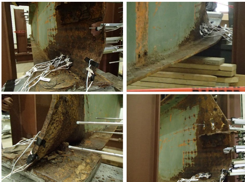
Figure 6.5: The residual deformation after unloading Specimen 1.
