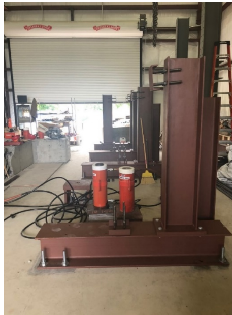
Figure 3.10: Experimental configuration in Aug. 2018; anchor block, floor beams, and lateral bracing in position.
