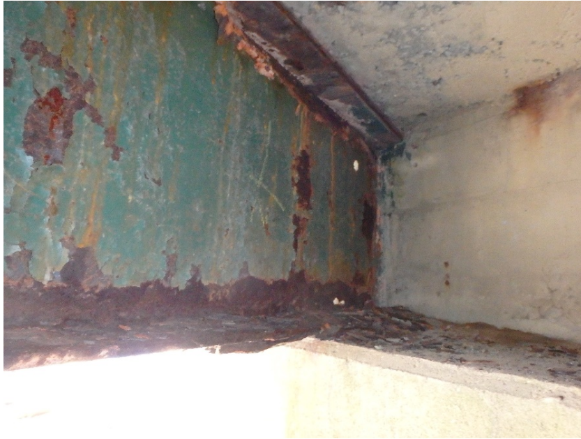
Figure 3.33: Bearing geometry of Charlemont bridge beams while in service.
