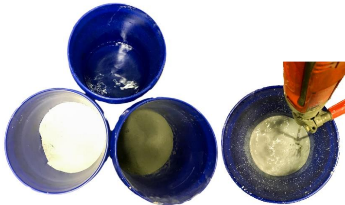
Figure A.3-6. Grout preparation for EMT specimens with buckets, paddle mixer, and power drill
