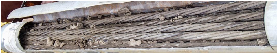
Figure A.4-9. Visual inspection of section 3 after water-blasting
