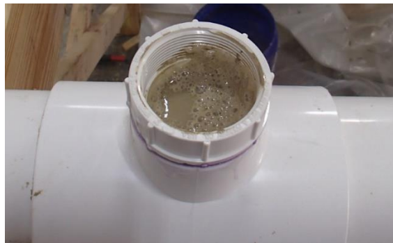
Figure 6-7. PVC tee through which grout was introduced
