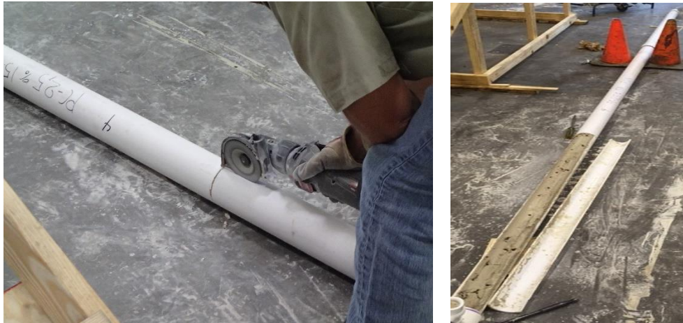
Figure A.3-8. Partial removal of PVC for inspection
