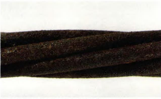
Photo 7. Strand surface before cleaning.
