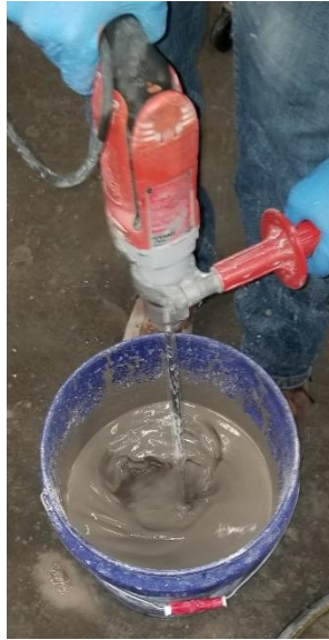
Figure 12-10. Grout mixing
