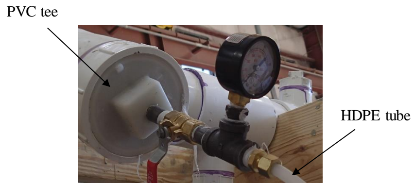
Figure 6-2. HDPE connection at PVC tee of inlet
