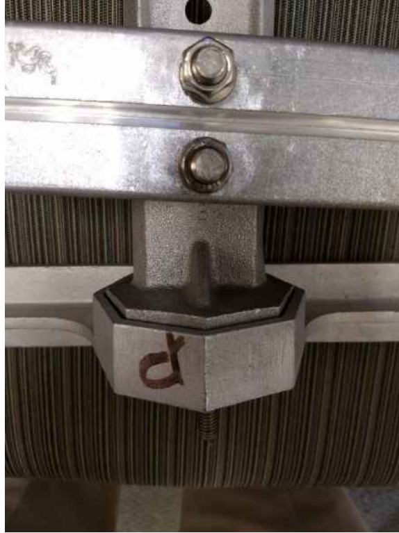
Figure 252: Connected octagon end with standard tri-stud adjustable hanger
