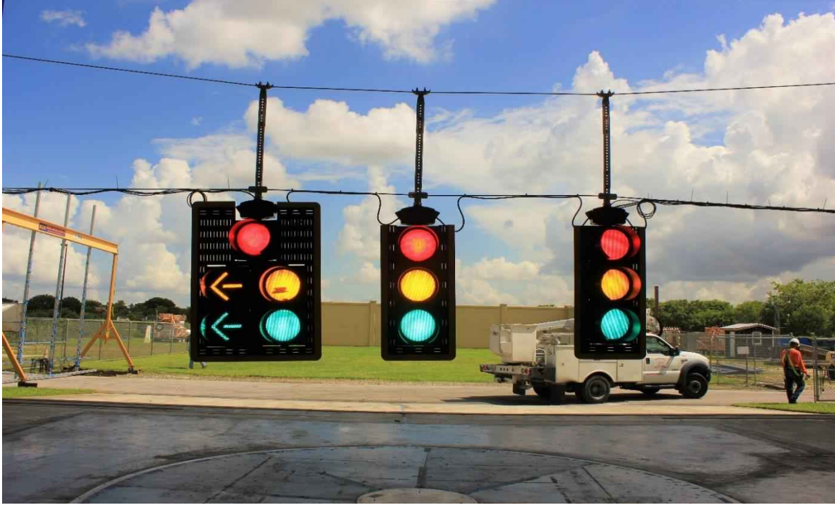
Figure 199: Traffic signals, hangers and span-wire
