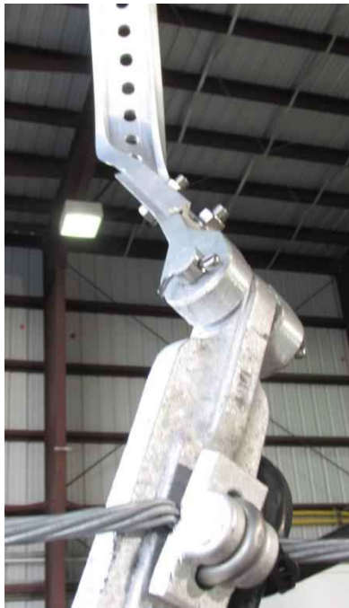
Figure 81: Twisted adjustable extension hanger for 5-section signal
