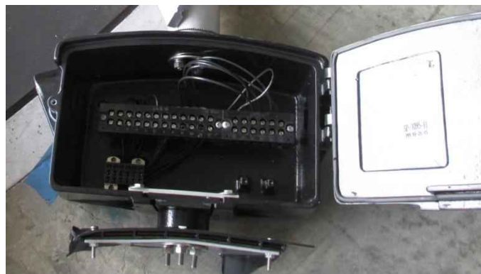
Figure 147: Disconnect box after completion of test and broken top portion of signal assembly
