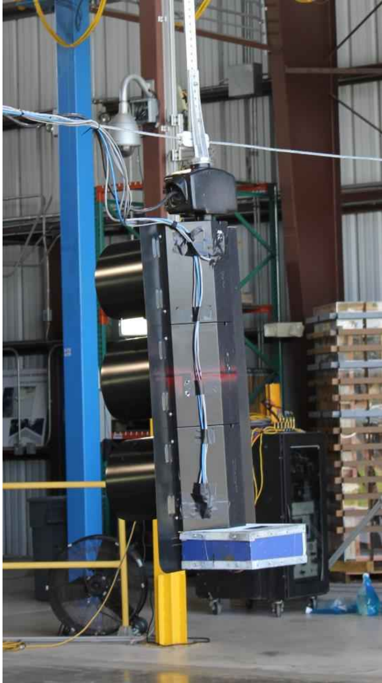
Figure 265: Close up of metal-box with iron-ball located at bottom of signal housing
