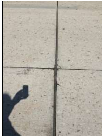
Figure 174. Corner cracking on rigid pavement.
