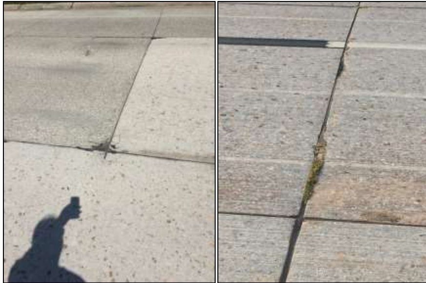
Figure 172. Spalling on rigid pavements.
