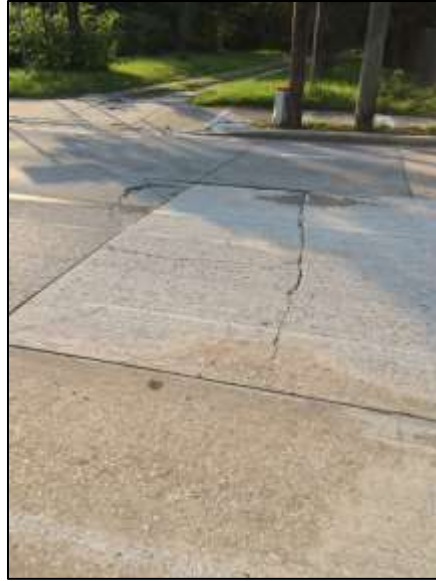
Figure 175. Shattered slab of rigid pavement.
