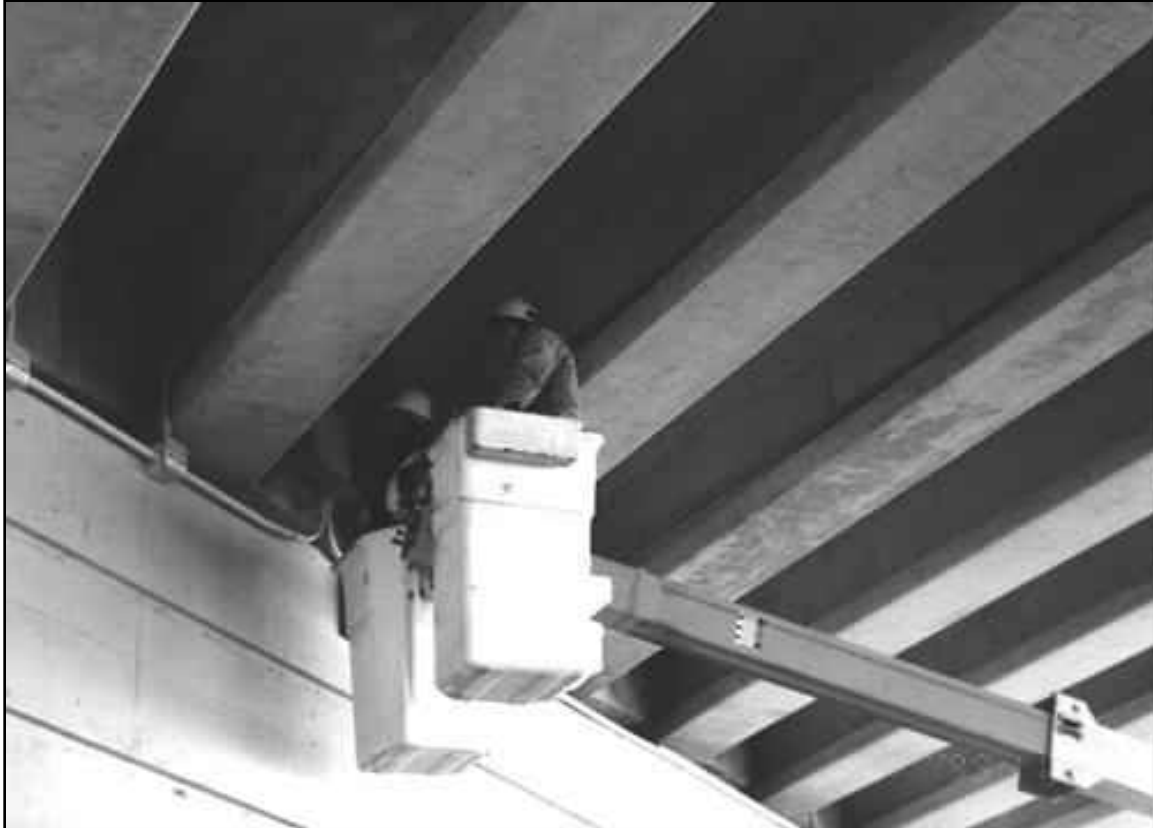
Figure 2.28: Beddington Trail Bridge, Calgary, Canada (ISIS Canada, 2009)
