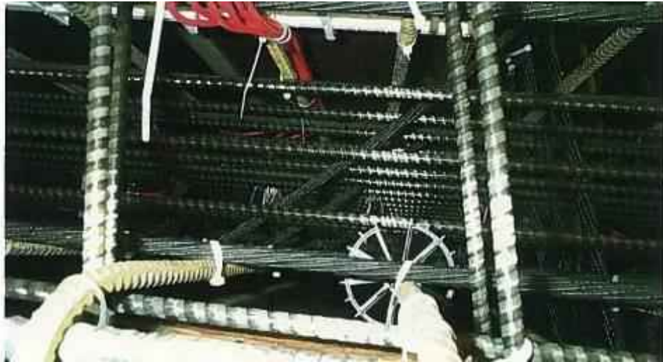
Figure 2.21: Instrumentation and CFRP reinforcing cage of one web (Grace et al. 2003).
