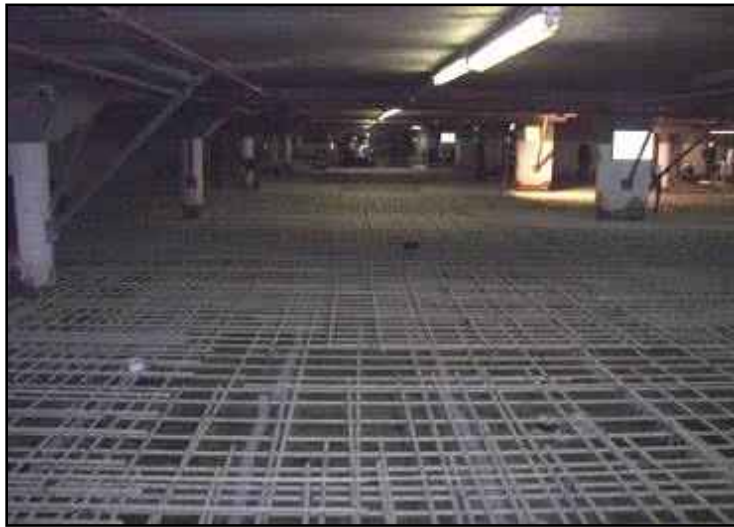
Figure 2.36: La Chancelière Parking Garage
