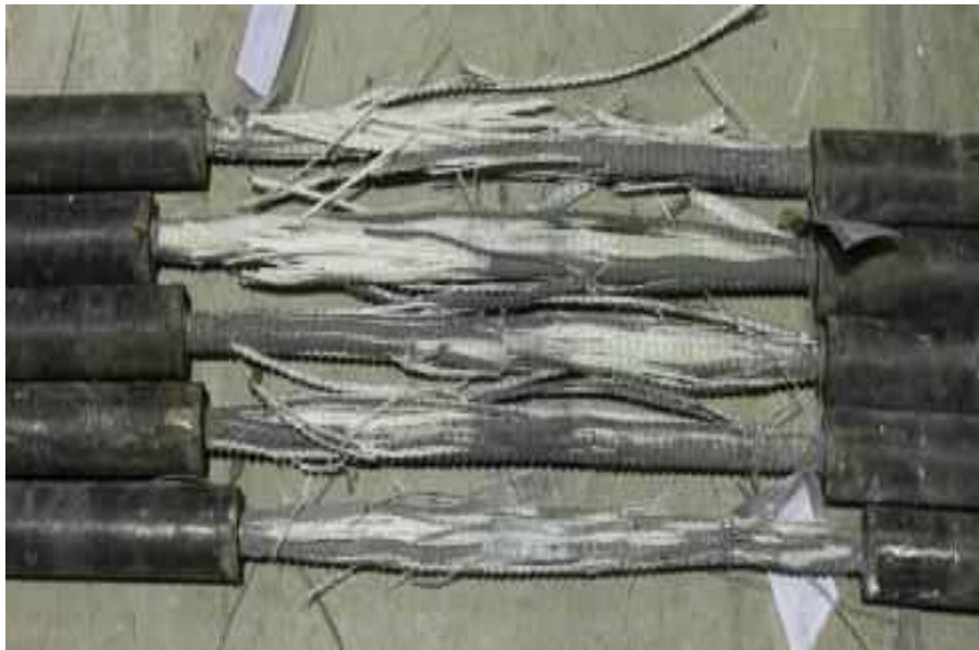
Figure 4.26: Typical mode of failure of vinyl ester GFRP bars
