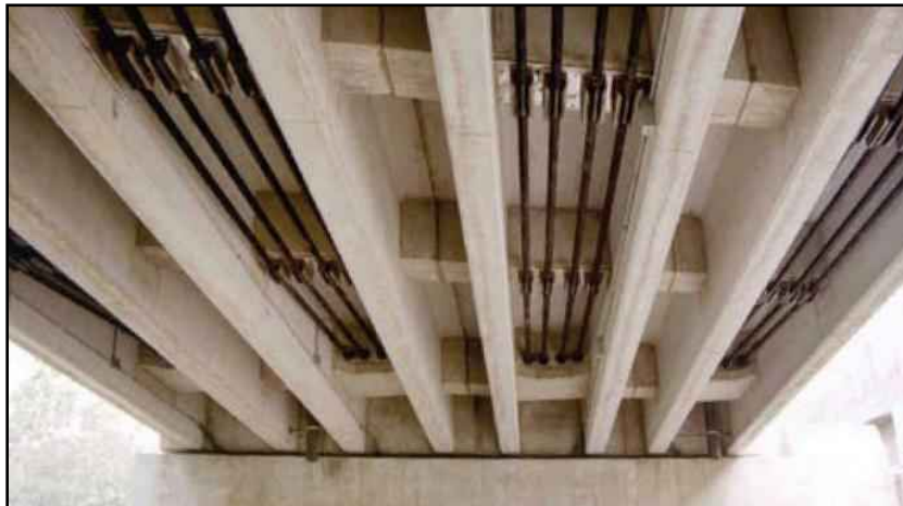
b) Installed double-T girders with external CFRP post-tensioning strands in place
