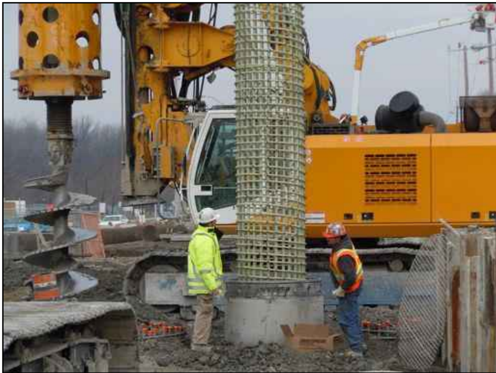
(b) Handling and lifting the GFRP soft eyes
