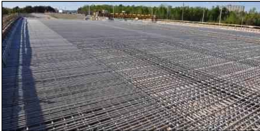
(c) Reinforcement of the bridge deck, 410 overpass bridge Quebec, Canada
