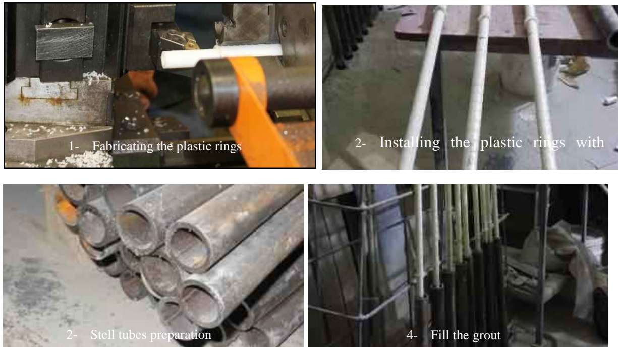
Figure 4.4: Preparation of the test GFRP bar specimens
