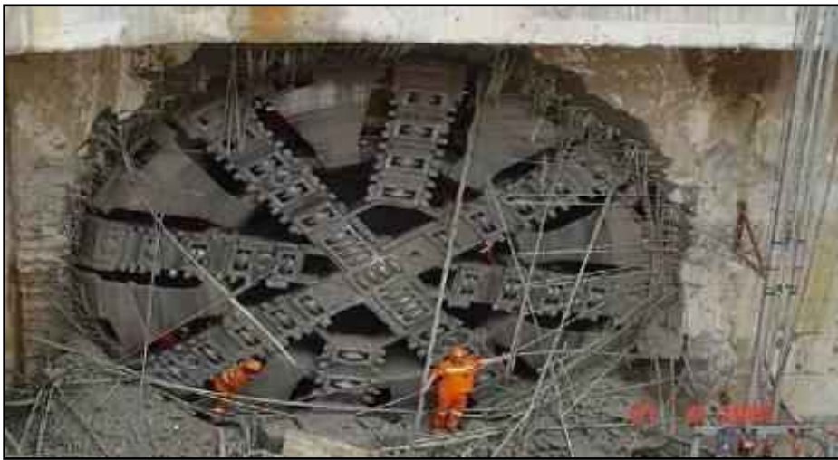
Figure 2.33: TBM cutting through FRP-reinforced concrete drilled shaft wall
