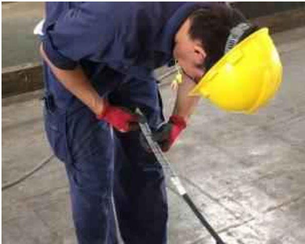
(c) Wrapping CFRP with buffer material
