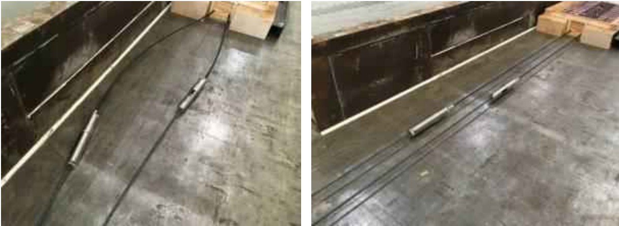
Figure 6.6: CFRP strands before and after tensioning.
