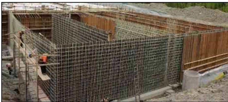
(a) FRP reinforcement bars of the vertical wall
