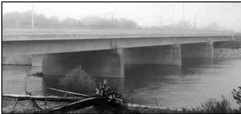
Figure 2.30: Taylor Bridge, Manitoba, Canada (ISIS Canada, 2009)
