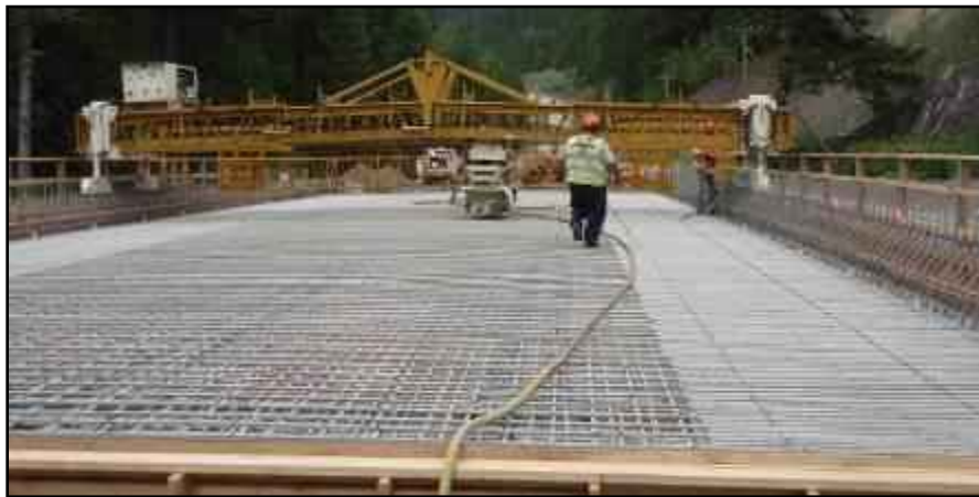
(a) FRP decks/app slabs/ barriers – Skagit River – BC MOT (2009)
