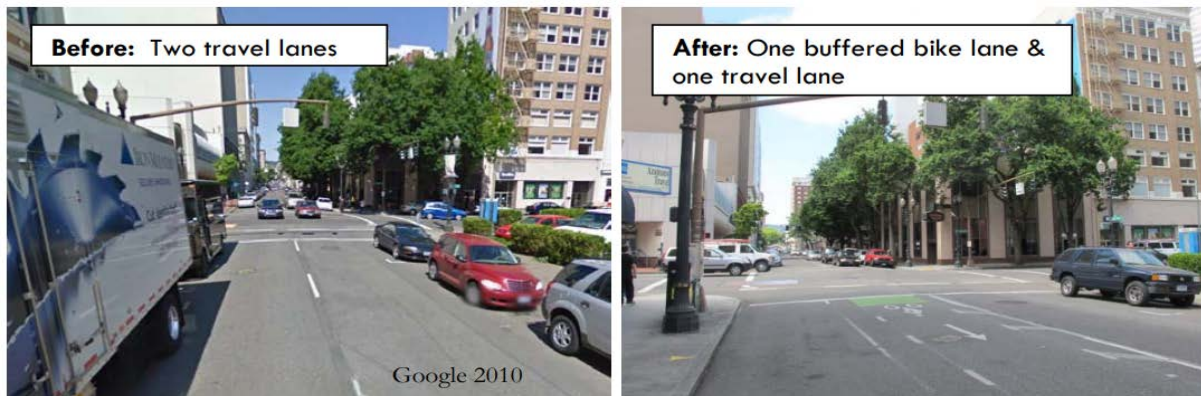
Figure 5-1. Stark St. at 4th Ave.: Street View Before and After Buffered Bike Lane Installation (Source: Monsere, McNeil & Dill, 2010)
