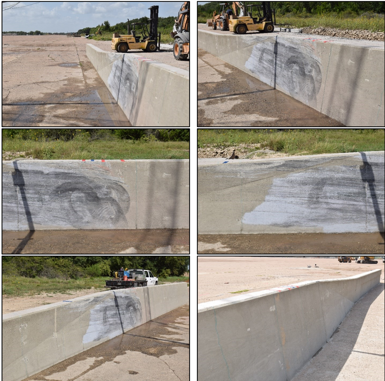
Figure 7.3. Transition after Test No. 469689-2-2.
