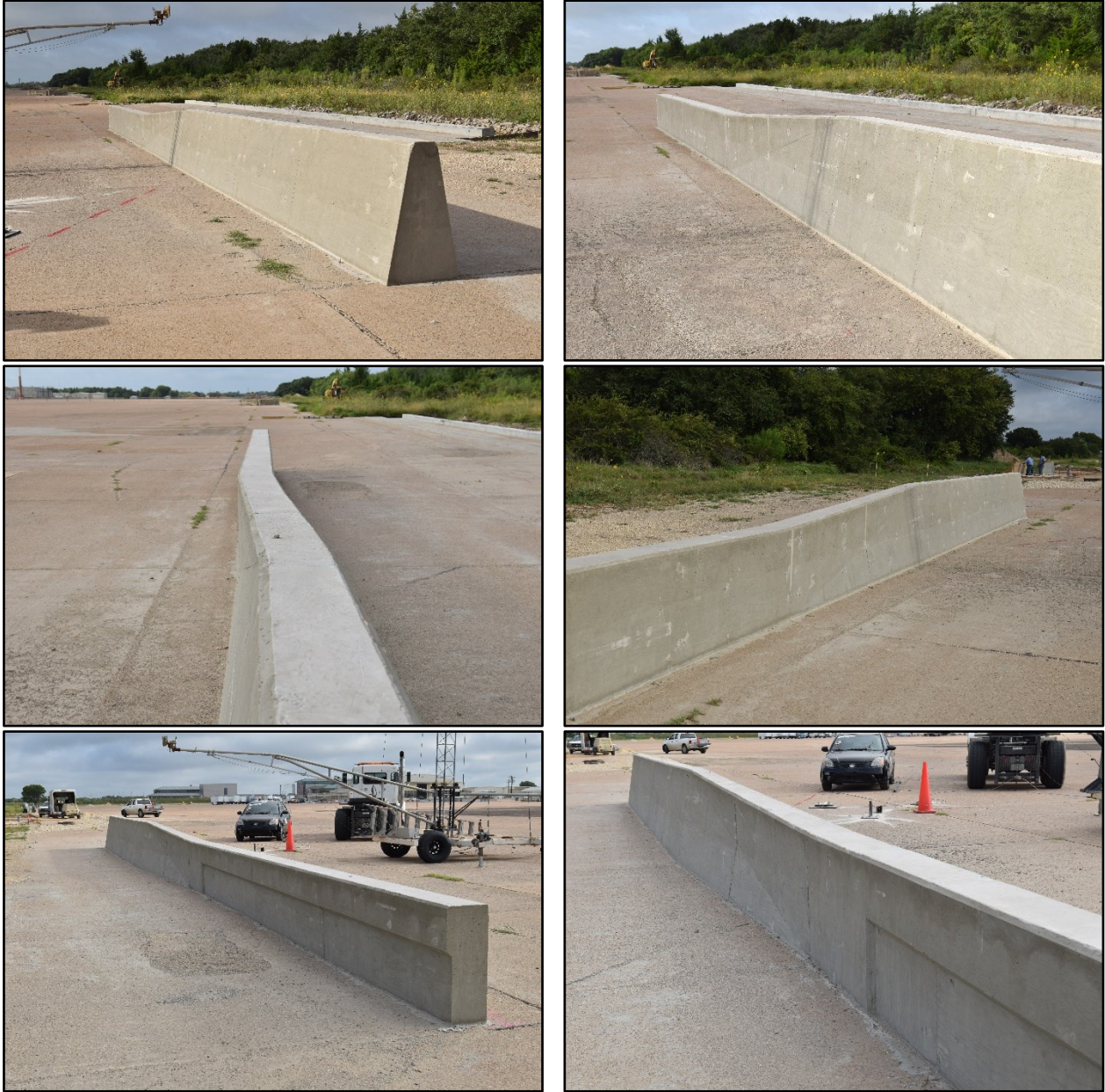
Figure 3.2. T221 Vertical Wall to SSCB Transition Prior to Testing.
