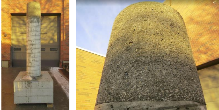
Figure 5.7. Completed precast column (left) and exposed aggregate finish (right)
