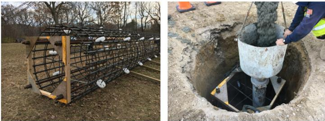
Figure 5.27. Construction of drilled shaft
