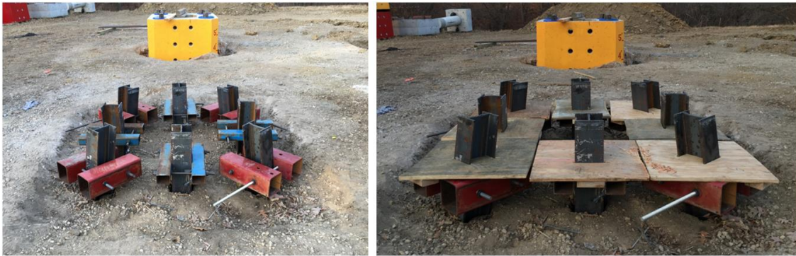
Figure 5.17. Friction collars and plywood seal-pads
