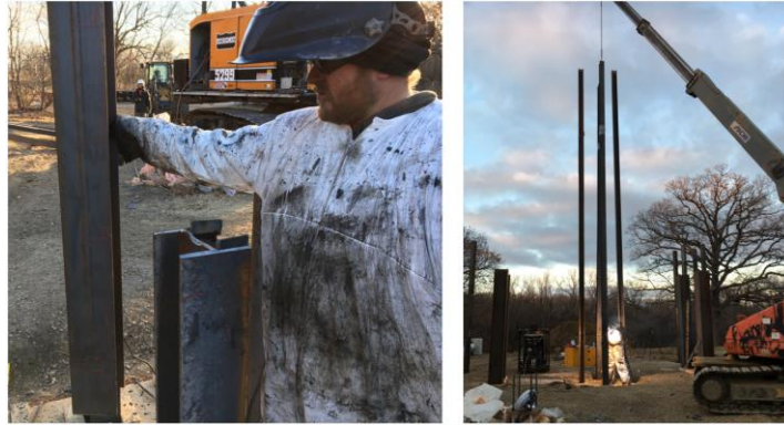
Figure 5.16. Weld-splicing piles
