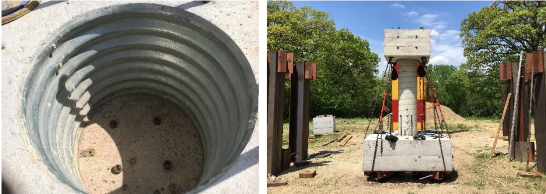
Figure 5.18. Nut shimmers underneath column (left) and temporary column bracing (right)
