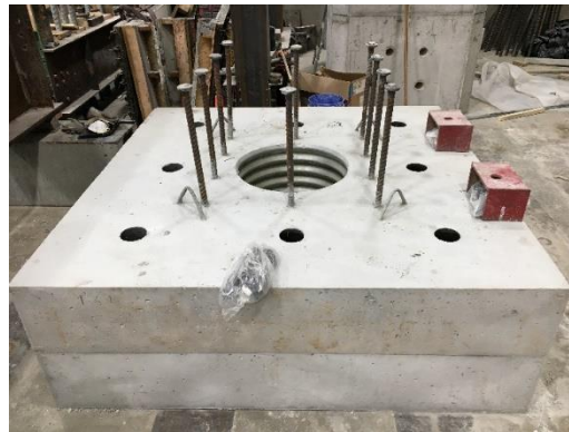
Figure 5.14. Completed precast pile cap
