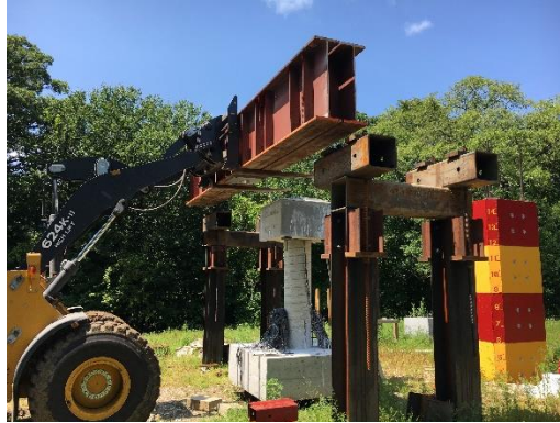
Figure 5.22. Placing main reaction beam
