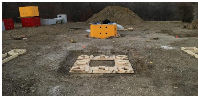
Figure 5.15. Driven pile template
