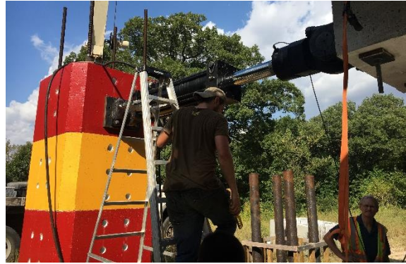
Figure 5.28. Lateral actuator attached on reaction column
