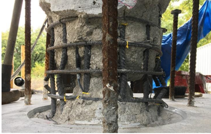
Figure 5.43. Column base at the end of Phase II
