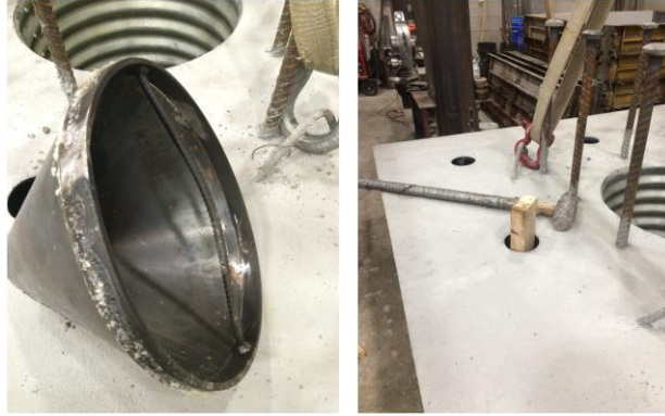
Figure 5.13. Taking out reusable reducers
