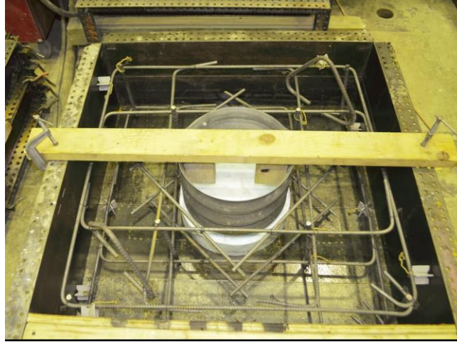
Figure 4.3. Reinforcing cage and CSP installation for foundation
