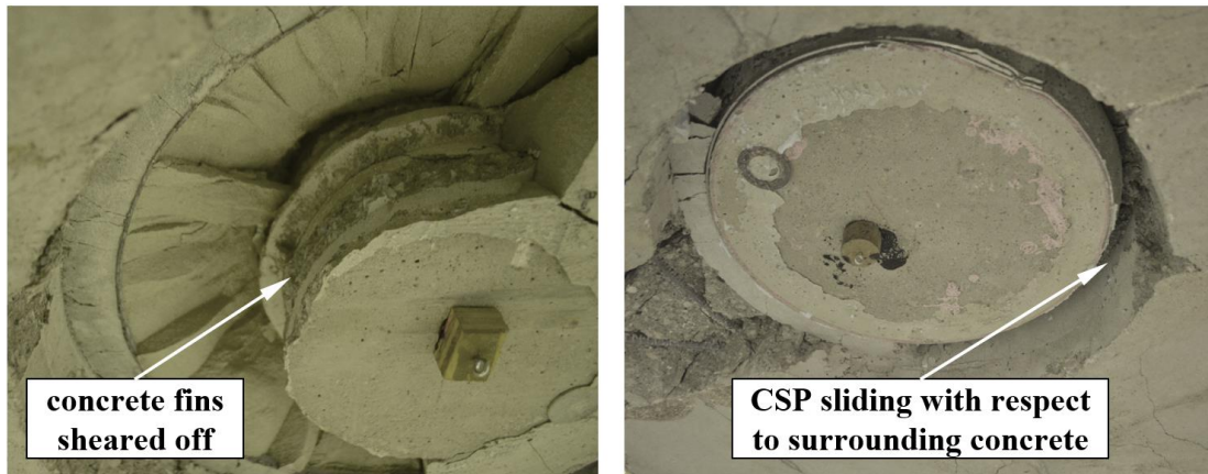
Figure 4.10. Failure modes of the specimens
