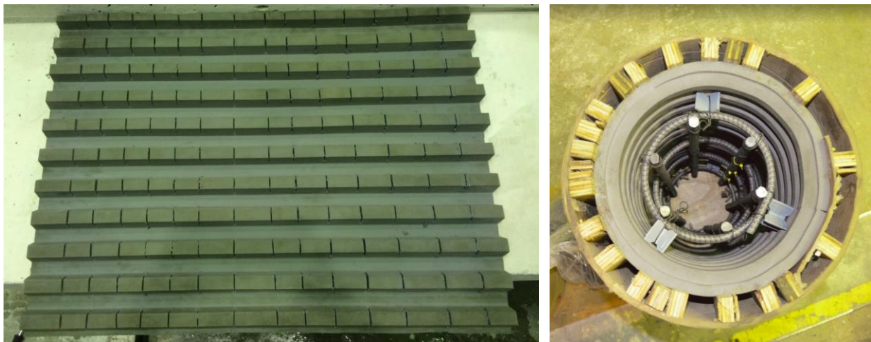
Figure 4.4. Form liner used to create fluted fins on the column
