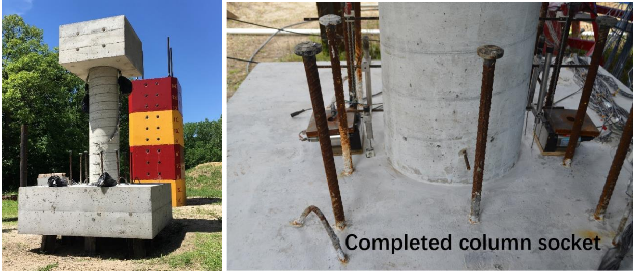
Figure 5.20. Completed test unit
