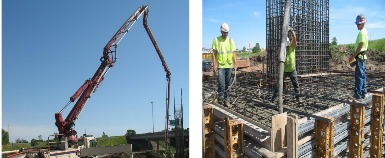
Figure 5.10. Pouring concrete using pump (left) and compaction using vibrator (right)
