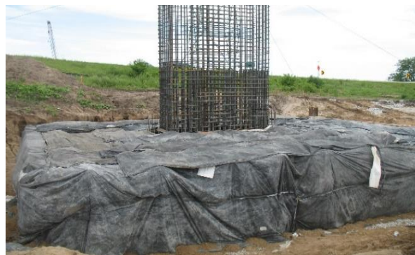
Figure 5.13. Insulation blanket over formwork
