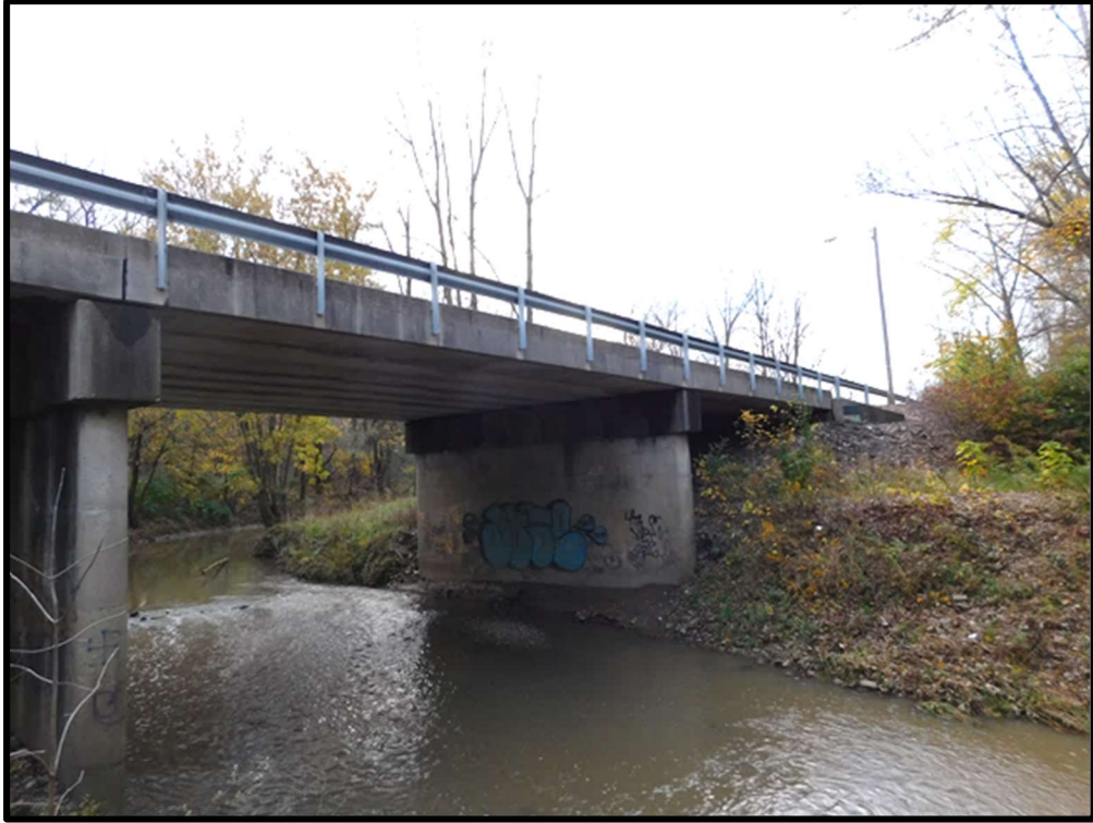
Figure 4.29 Main Street Bridge.
