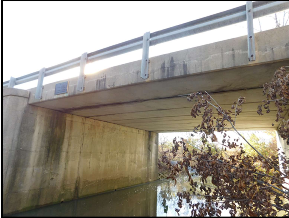
Figure 4.24 Beal-Taylor Ditch Bridge.
