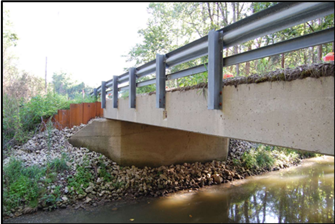
Figure 4.3 Pond creek bridge.
