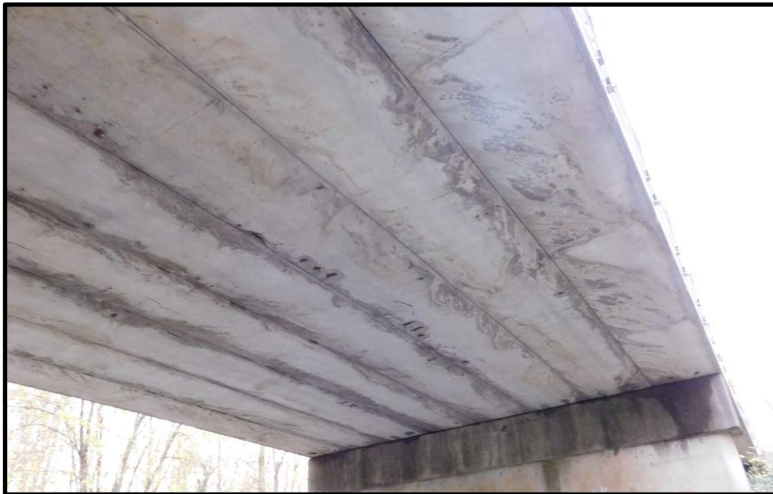
Figure 4.33 Middle span of Main Street Bridge
