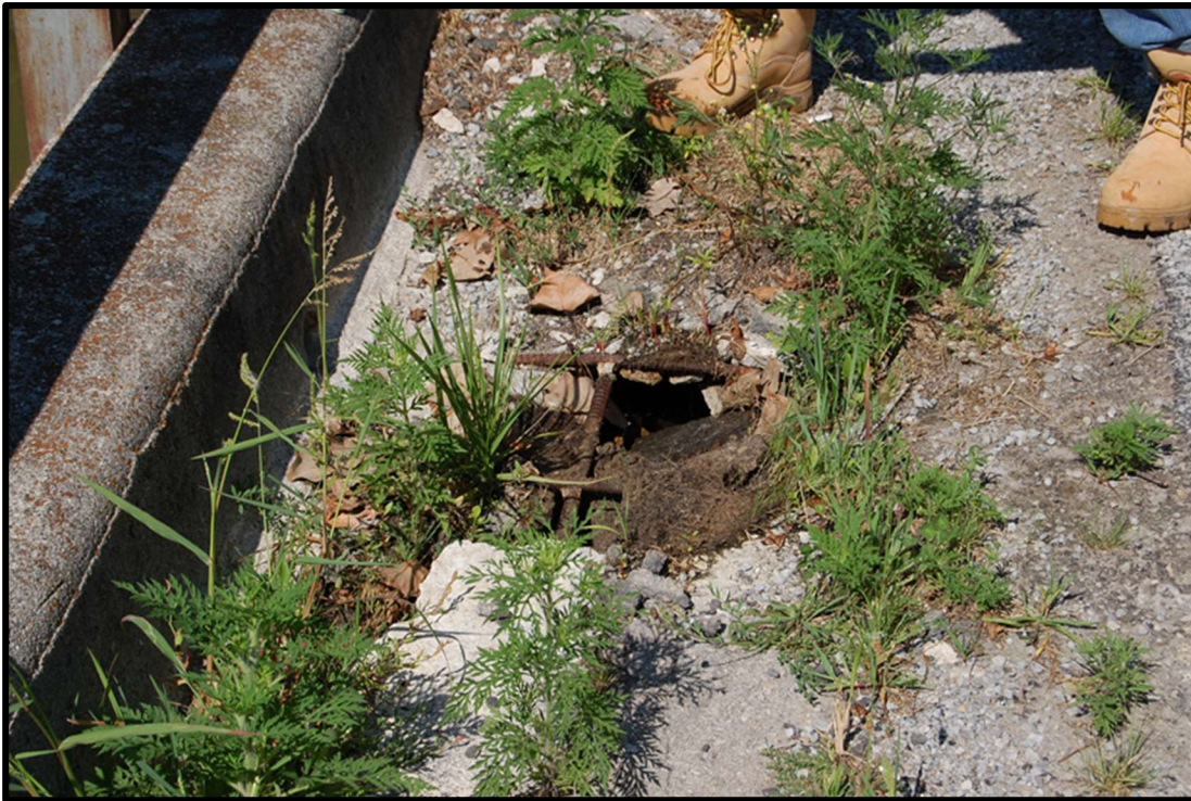
Figure 4.47 Opening in top flange of exterior beam (Rock Creek).
