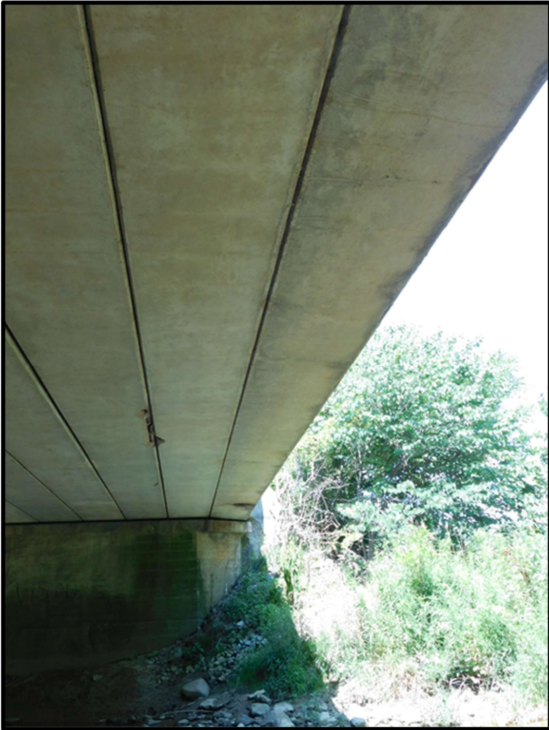
Figure 4.46 Rotation of exterior beam (Clear Creek).
