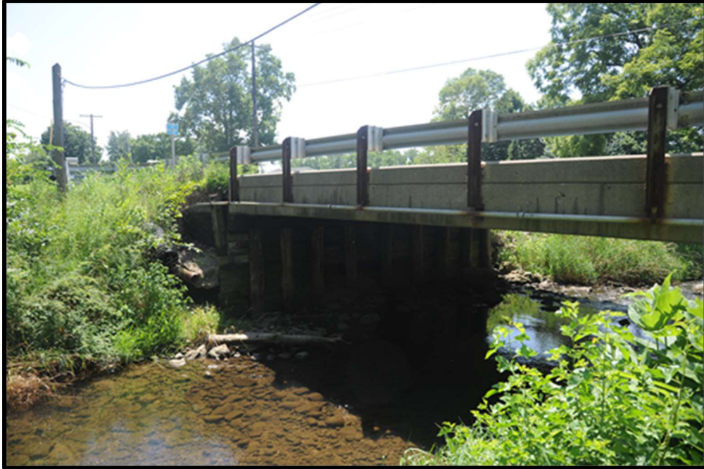
Figure 4.18 Yellow Creek Bridge.
