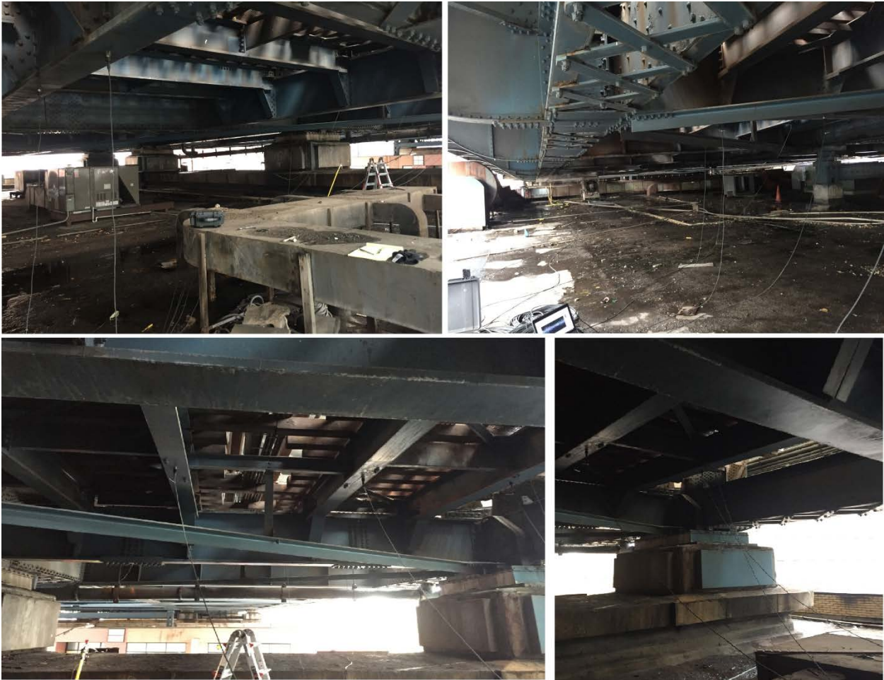
Figure 8 Accelerometer locations (southbound)
