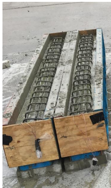
Figure 5-9: Substrate casting (of the \frac{2}{3} upper beam height) in inverted position
