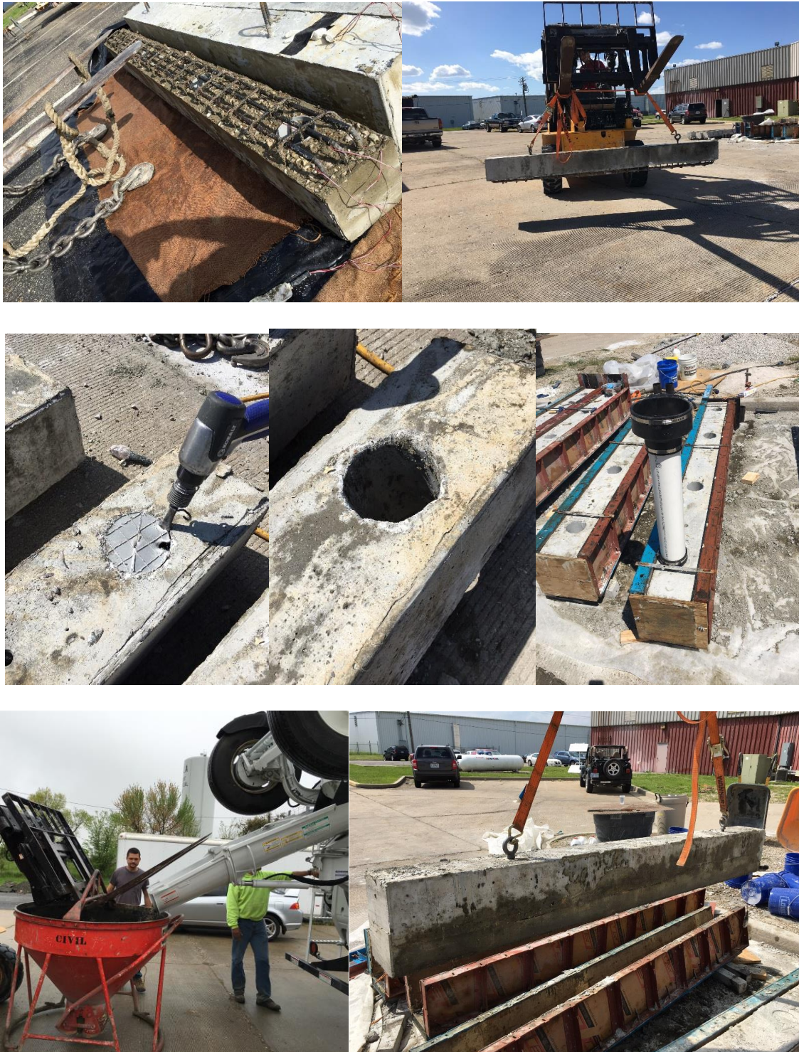
Figure 5-11: Repairing of CVC Beams using FR-SCC
