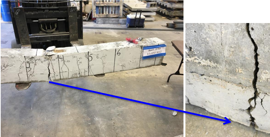
Figure 5-19: Repaired beam after loading up to failure
