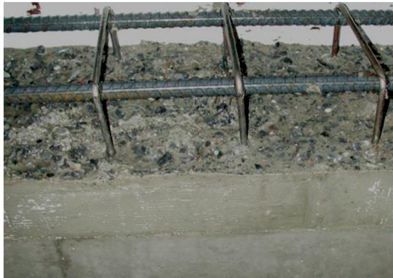
Figure 2-55: Roughened surface of base concrete before casting repair materials
