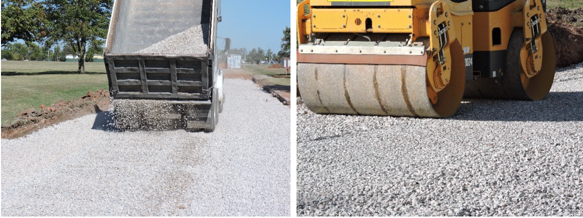
Figure 10-4. Installation (l) and Compaction (r) of Pavement Aggregate Base
