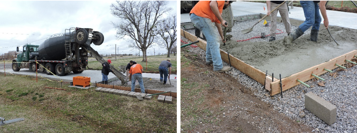
Figure 10-12. Concrete Placement (l) and Consolidation (r)
