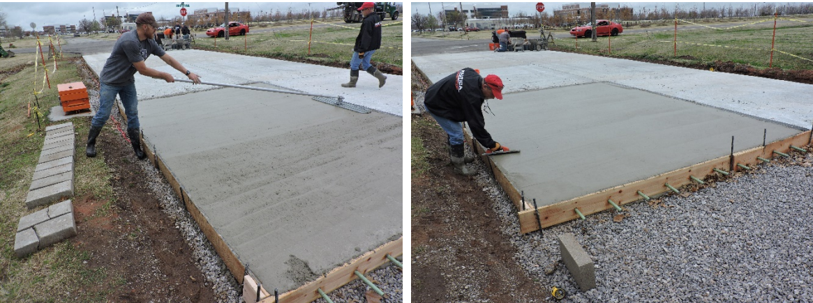
Figure 10-13. Concrete Floating (l) and Finishing (r)
