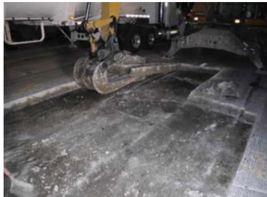
Figure 7: Excavator Method for removal of existing pavement (NPCA, 2017).
