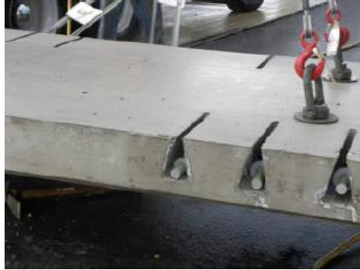
Figure 11: SHRP2 standard narrow-mouth dowel system (from Tayabji and Brink, 2015).
