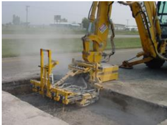
Figure 19: Gang drill- EZ Drill Model 210 used for pre-drilling holes for dowel insertion using narrow mouthed dowel connect (Concrete Products, 2017)
