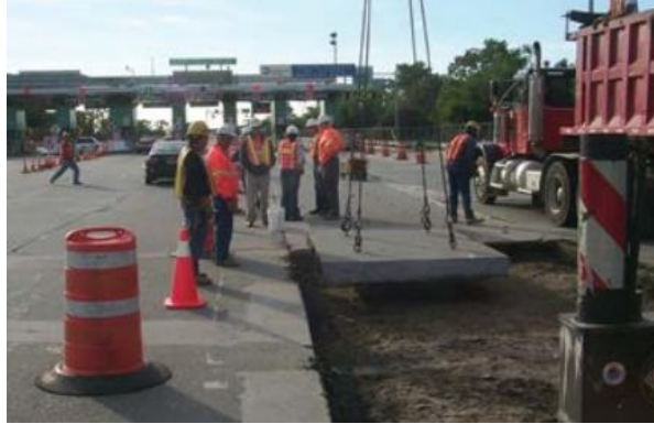
Figure 6: Lift out method for removal of existing pavement. (NPCA, 2017)
