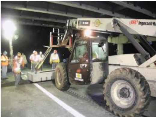
Figure 4: Fork truck installing precast panel beneath an overpass (NPCA, 2017).
