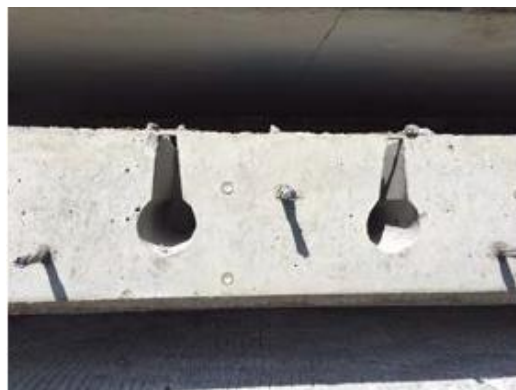
Figure 13: Caltrans standard teardrop-shaped narrow-mouth system (from Tayabji and Brink, 2015).
