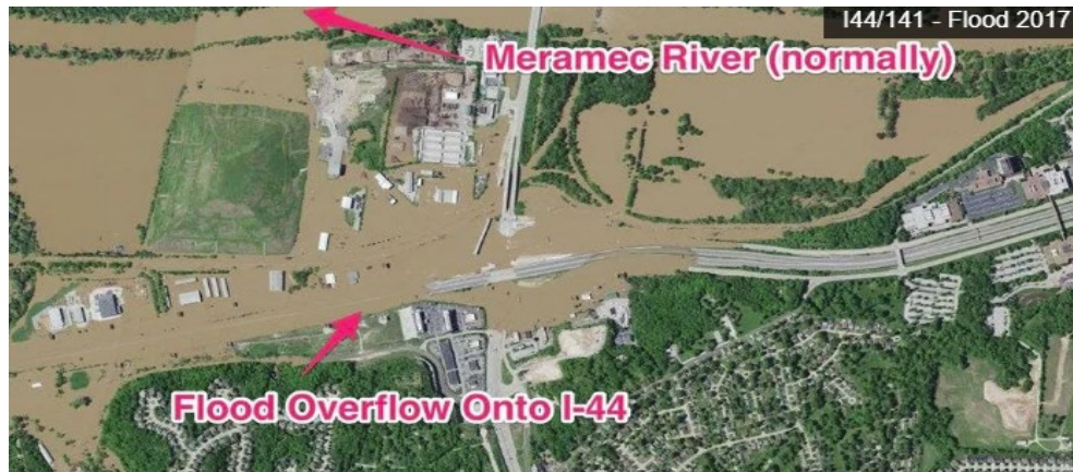
Figure 3.2 Intersection of I-44 and 141 during Meramec River floods in 2017 (Photos: Before & After Meramec River Flooding)
