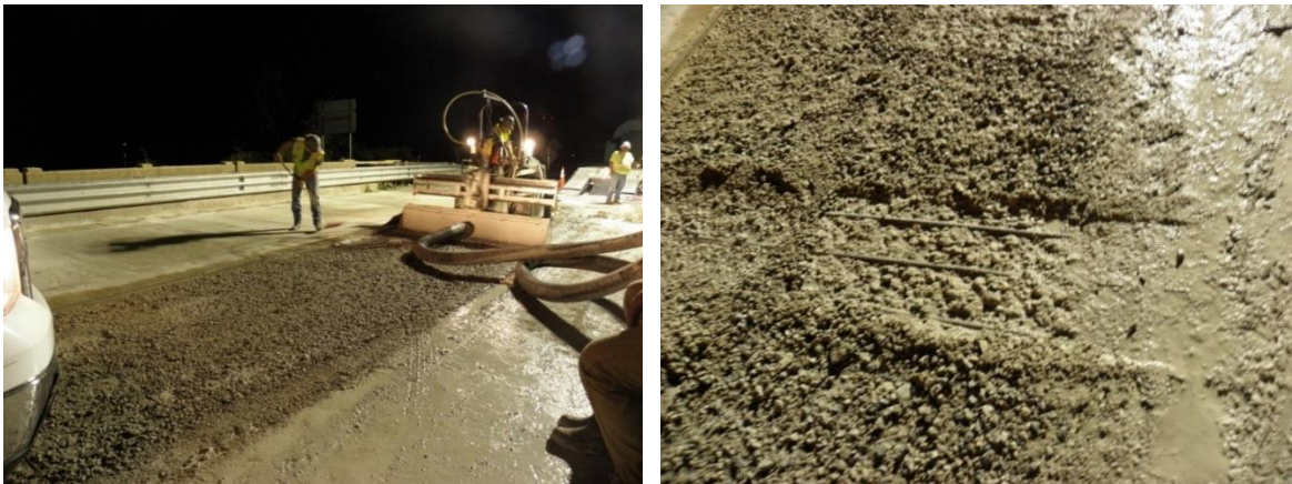
Figure 1: Hydrodemolition Equipment (left) and Post Hydrodemolition Surface (right)
