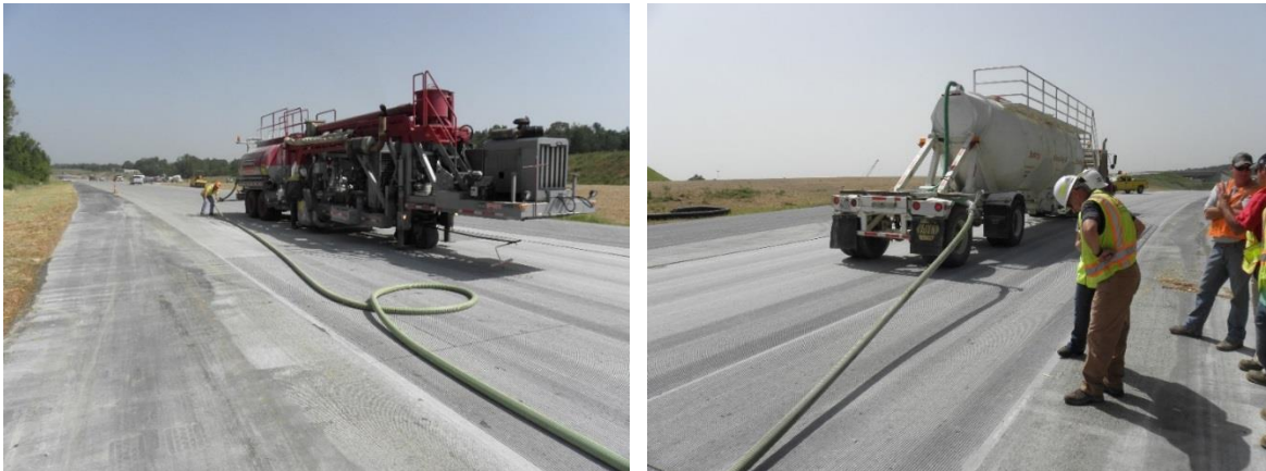
Figure 2: Diamond Grinding Machine (left) and Water Supply Tank (right)
