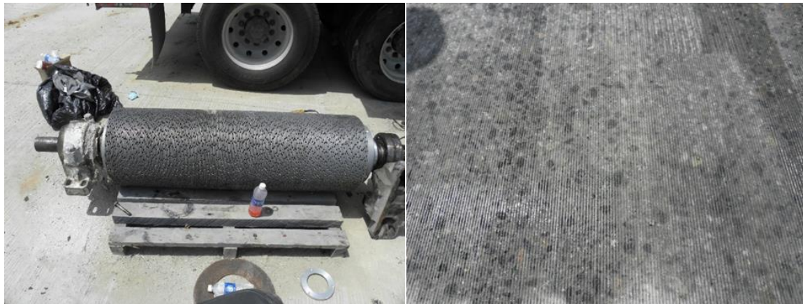
Figure 3: Diamond Grinding Saw (left) and Typical Grinded Section (right)
