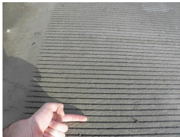
Figure 6: Typical Grooved Pavement Section
