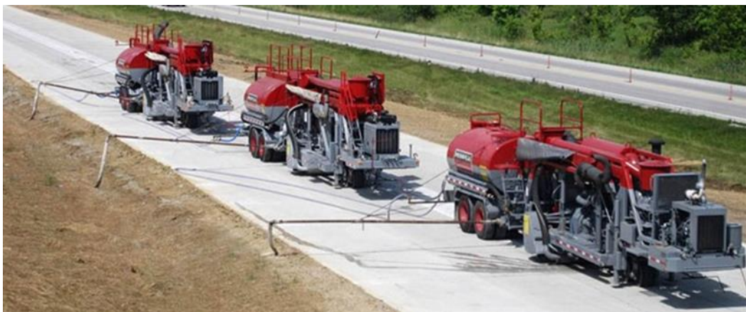
Figure 7: Side Slope Slurry Spreading (Penhall 2014)
