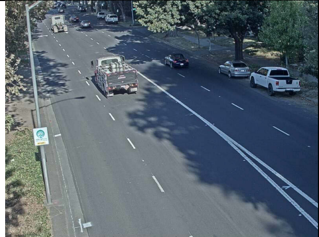
US 50 WB 10th St exit ramp
