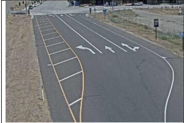
US 50 WB South River Rd exit ramp
