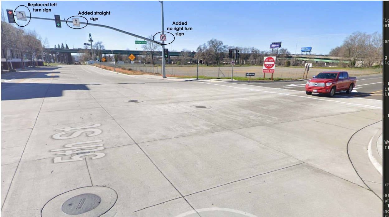
Figure 4.39: Caltrans' sign modifications and additions for southbound 5th Street on the south side of the intersection at the South River Road exit ramp. Image courtesy of Google Street View.
