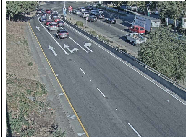
US 50 WB 16th St exit ramp
