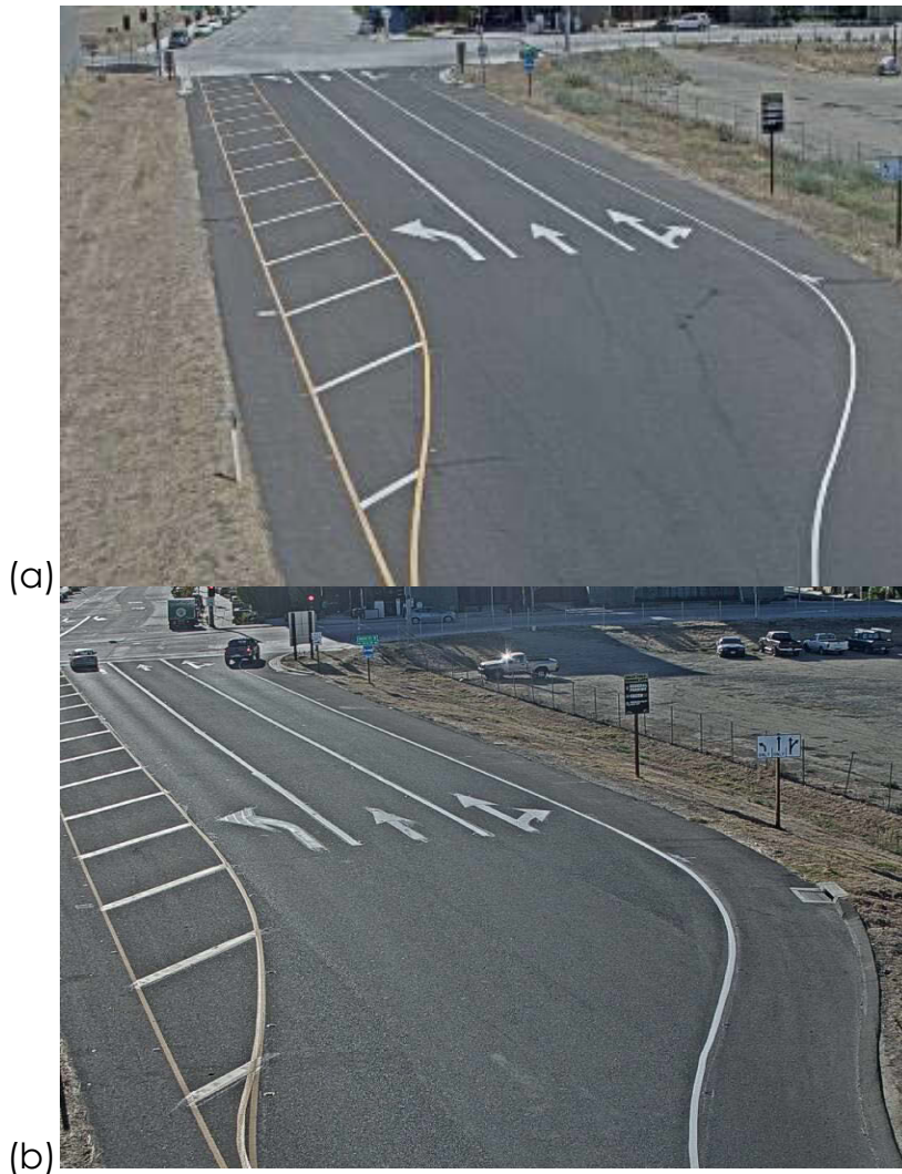
Figure 3.7: Effect of pole twist on the US 50 WB South River Road exit ramp WWD monitoring installation. (a) Camera FOV immediately after installation. (b) Camera FOV three months after installation.
