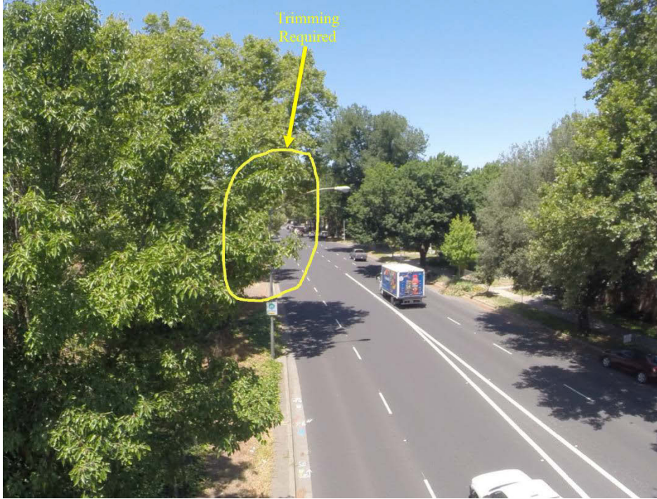
Figure 3.2: Example of tree trimming required to provide better camera FOV (US 50 WB 10 th St exit)
