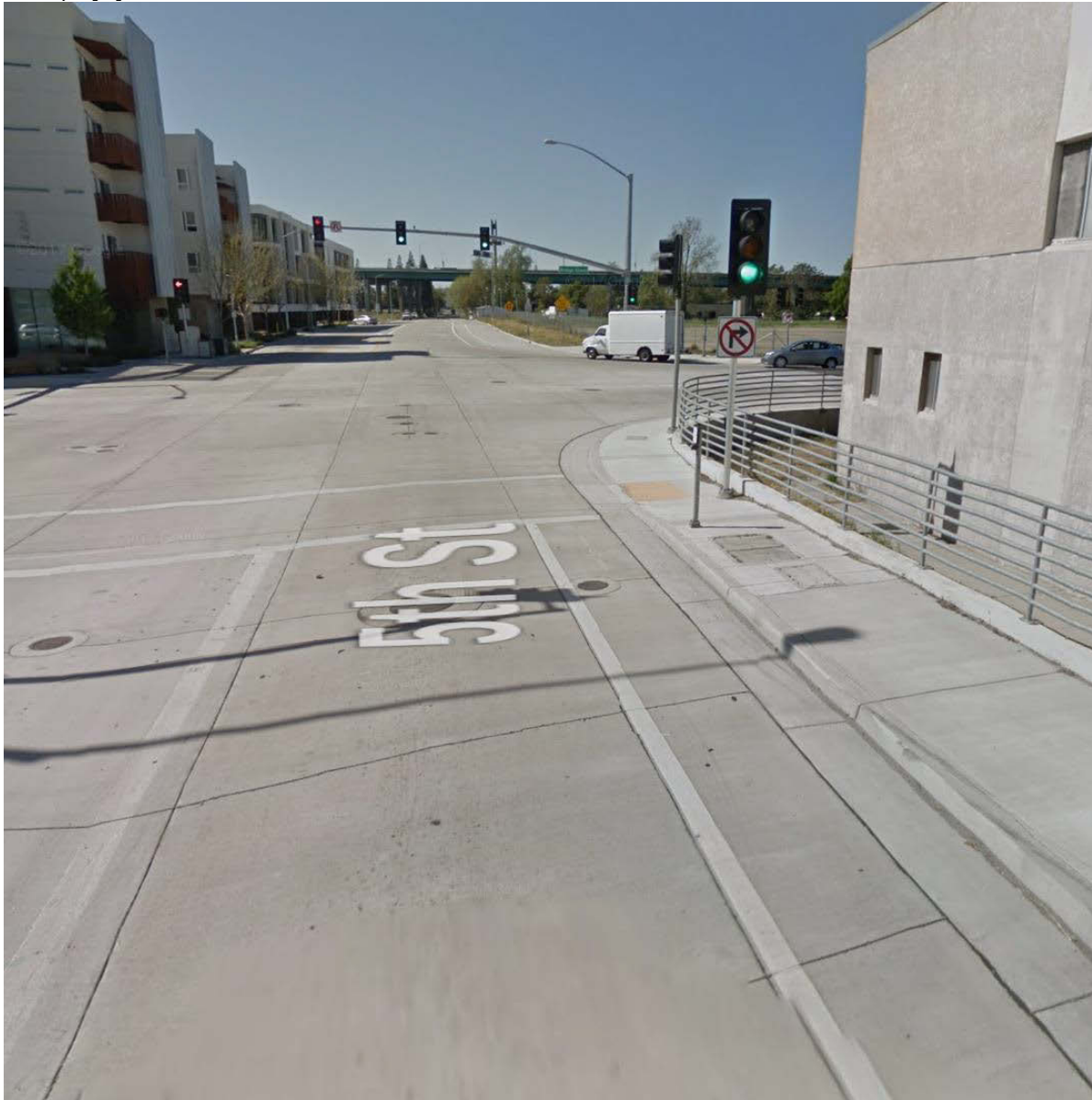
Figure 4.23: View of the approach from the north to the South River Road exit ramp. A right turn would lead to a WWD event. Image courtesy of Google Street View.
