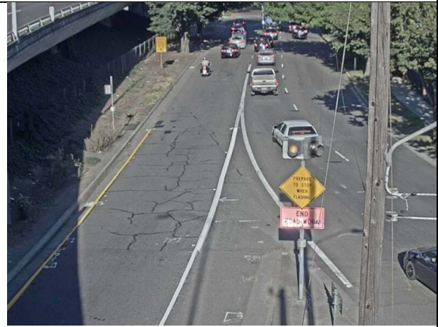
US 50 WB 26th St exit ramp
