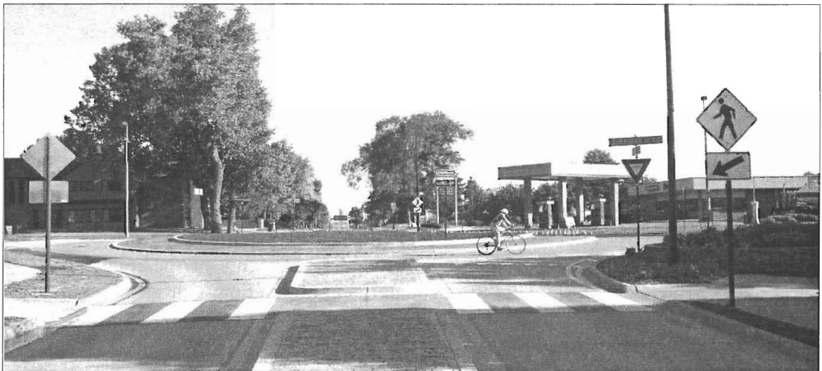
FIGURE 1B Example of Central Island with Clear Sight Line Cross View (Sheridan Boulevard and 33 rd Street Intersection, Lincoln, NE)
