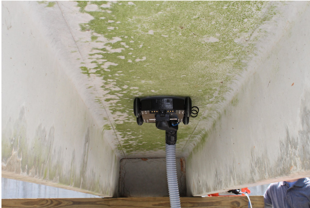
Figure 3.21. RTT vacuum prototype operating under double-tee concrete girder
