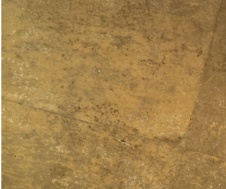
Figure 4.11. Image taken from drone recording (overhead view) of cracks in bridge deck
