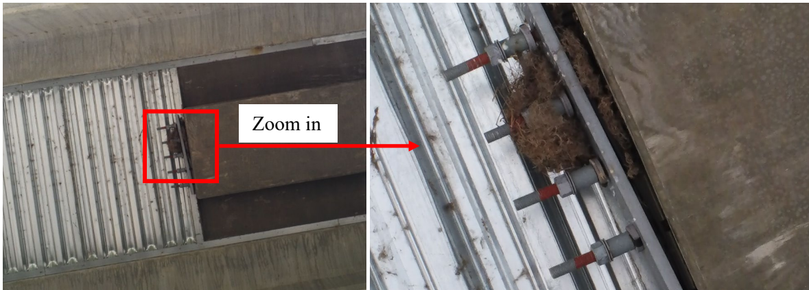
Figure 4.21. Image of superstructure with loose baseplate (taken by Parrot Anafi drone)
