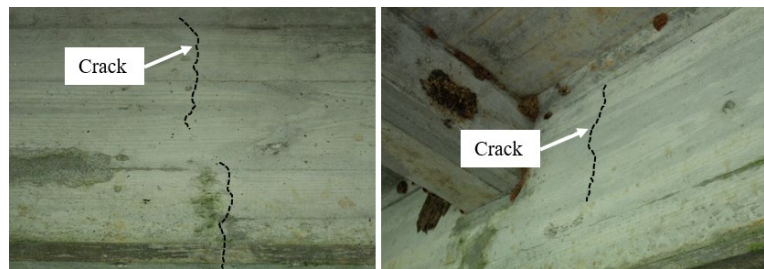
Figure 5.3. Visible cracks near to the midspan of interior girders
