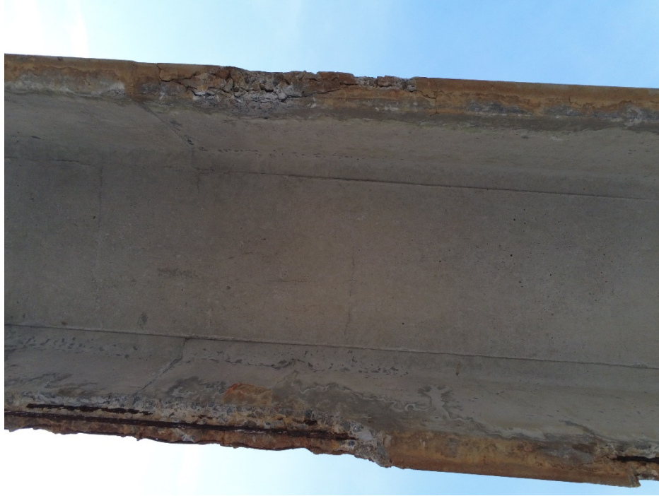
Figure 3.7. View from below double-tee girders
