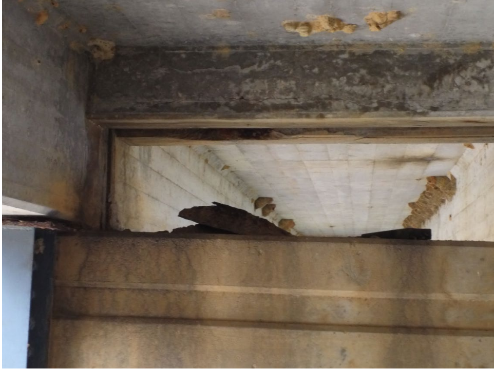
Figure 4.6. Cracking and corrosion (interior girder)
