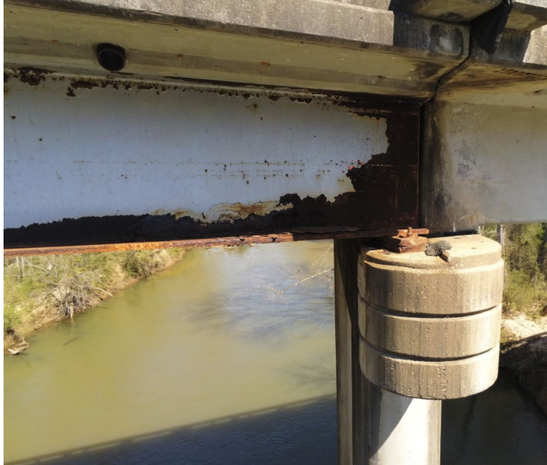
Figure 4.9. Drone image of corrosion on steel superstructure
