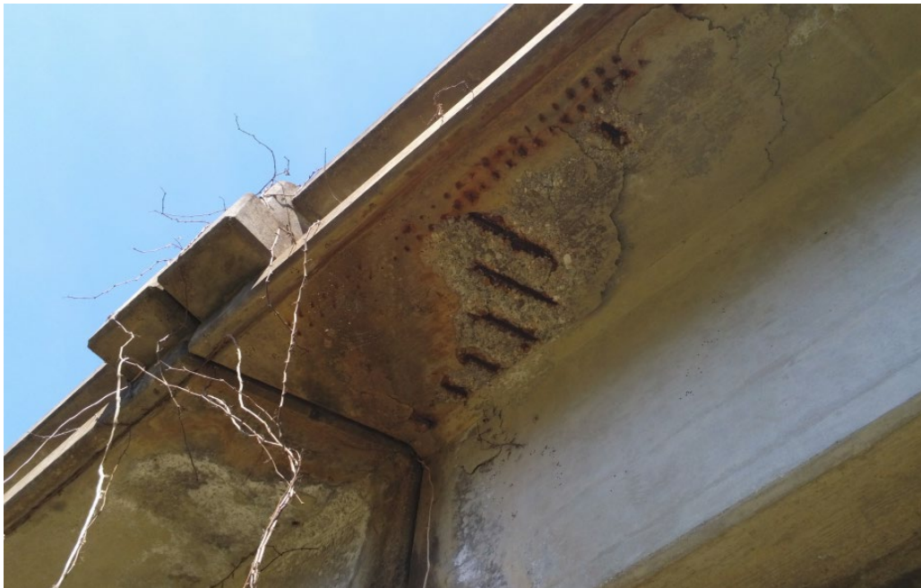
Figure 4.10. Delamination and crack development in SC HWY 105 Pacolet River Bridge
