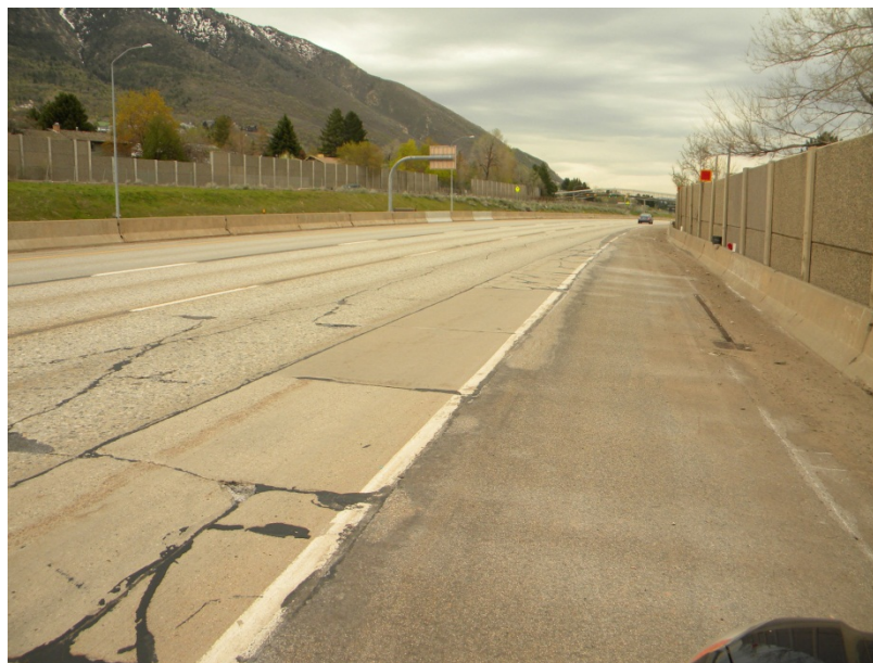
Figure 3. Southbound project view showing three lanes, merge area, and shoulder.
