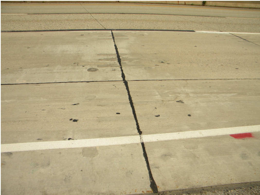
Figure 31. Transverse joint with grout-filled dowel bar slots.
