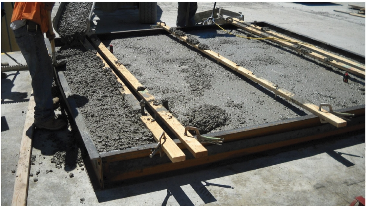
Figure 15. Pouring concrete in form to precast the panel.
