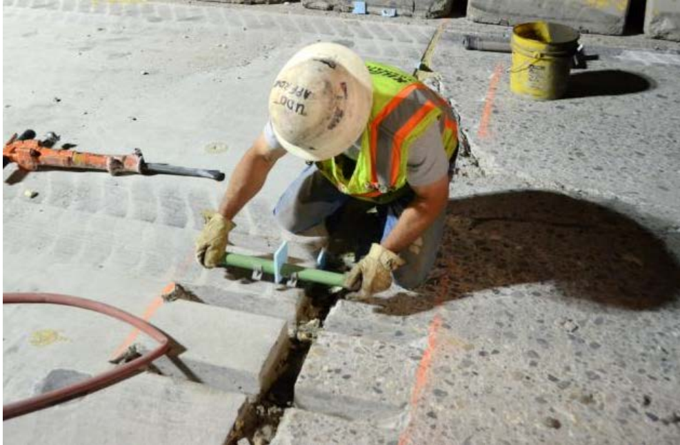
Figure 30. Placement of dowel bars into dowel slot.
