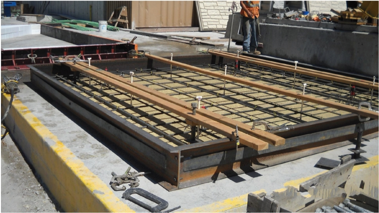
Figure 14. Completed form ready for concrete pour.
