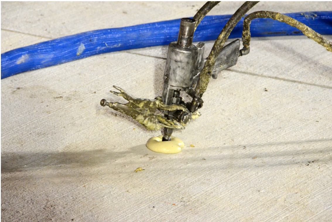
Figure 29. Urethane grout injection closeup.
