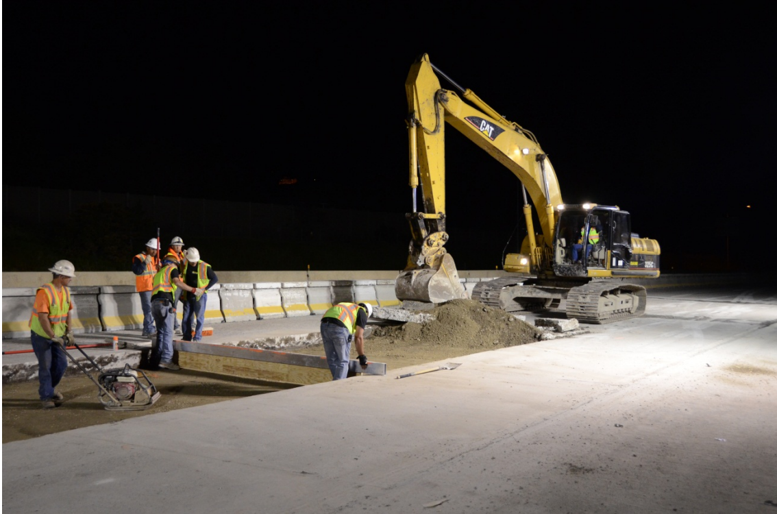
Figure 20. Placing and compacting the base course fill material.
