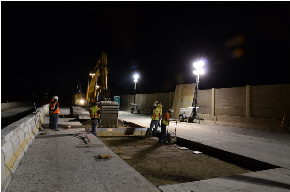
Figure 21. Leveling plates placed directly on top of the compacted base.
