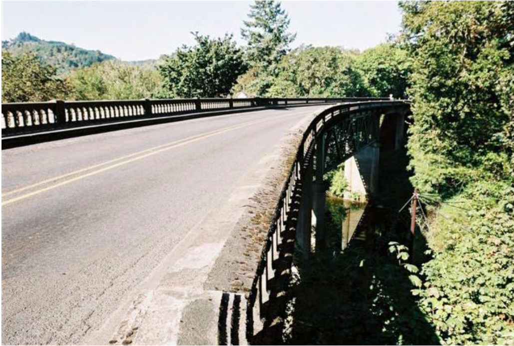
Figure 6. Old bridge over Elk Creek near Elkton (crossing 1).
