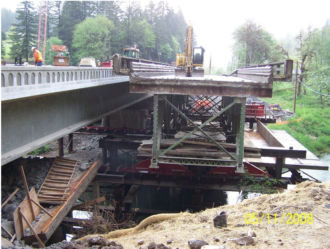
Figure B-1. Old and new superstructures side by side for crossing 4.
