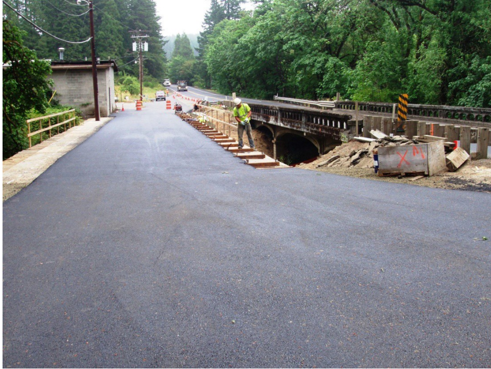
Figure 26. View of the temporary and old bridges looking east.
