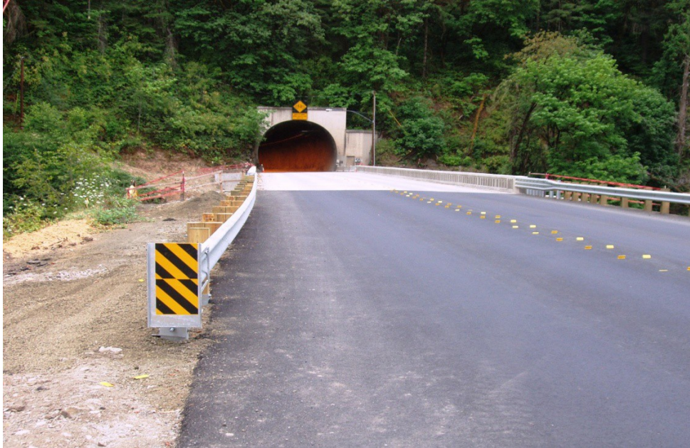
Figure 23. Completed crossing 4 after opening to traffic.
