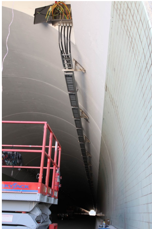
Figure 12. Photo. Installation of LED lighting system.
