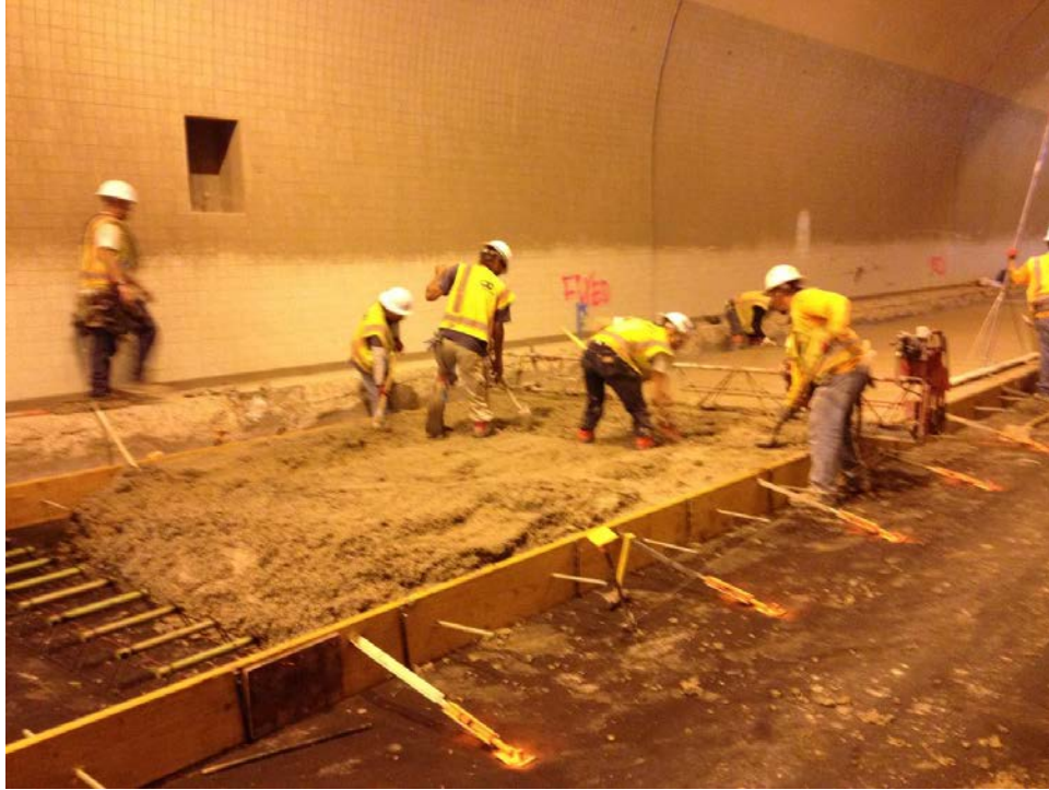
Figure 11. Photo. Reconstruction of rigid pavement structure within Carlin Tunnels.
