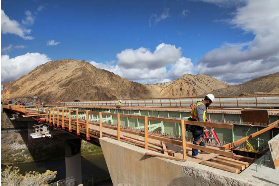
Figure 13. Photo. Bridge rehabilitation.
