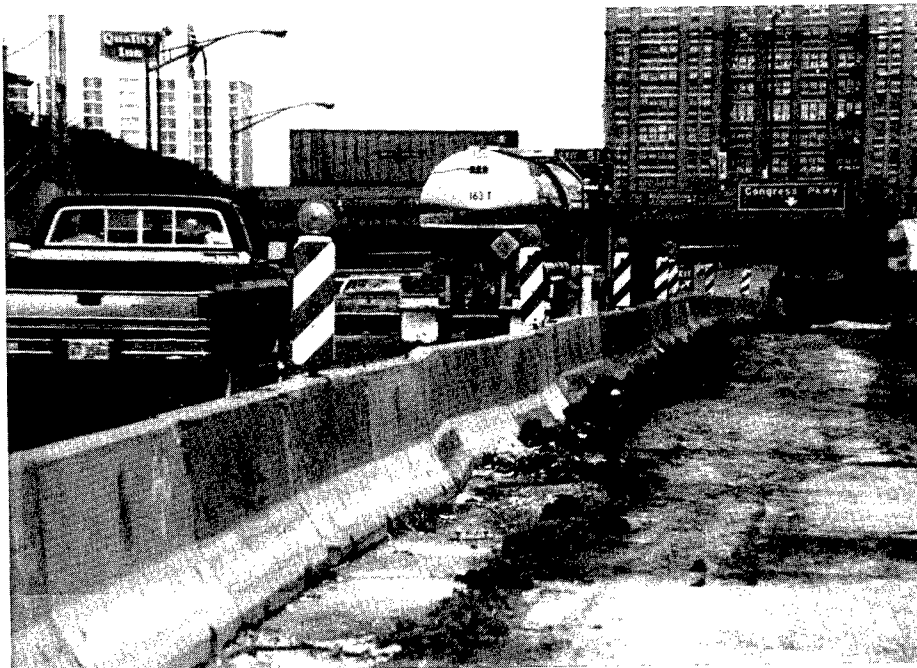
Figure 13. Combined use of warning lights and vertical panels
