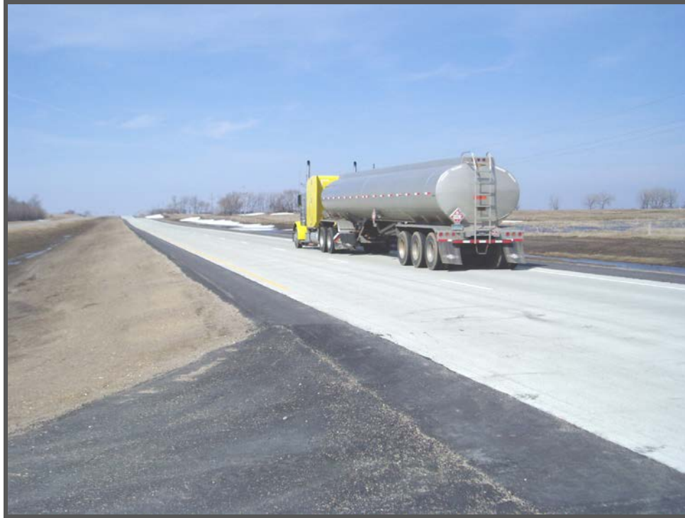
Figure 7. Completed whitetopped pavement.
