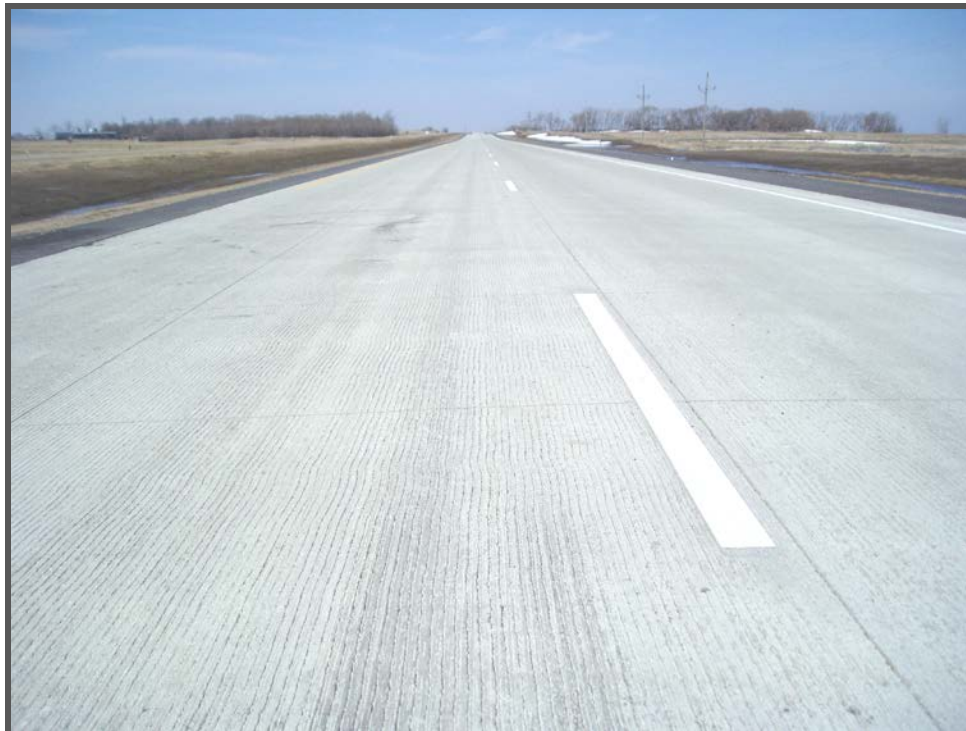
Figure 8. Closeup of the completed whitetopping showing the longitudinally tined surface texture and sawcut joints.
